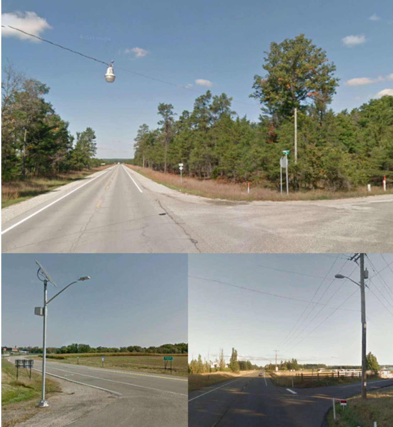
Figure 4. Photo. Examples of single luminaire intersection lighting (Image credit: Google Earth™ Mapping Service). (21)
