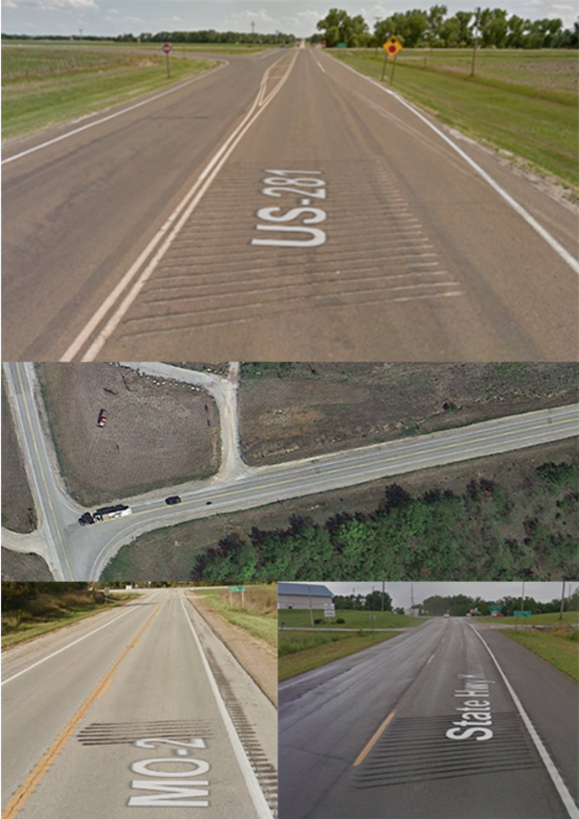
Figure 8. Photo. Examples of transverse rumble strips placement (Image credit: Google Earth™ Mapping Service). (21)
