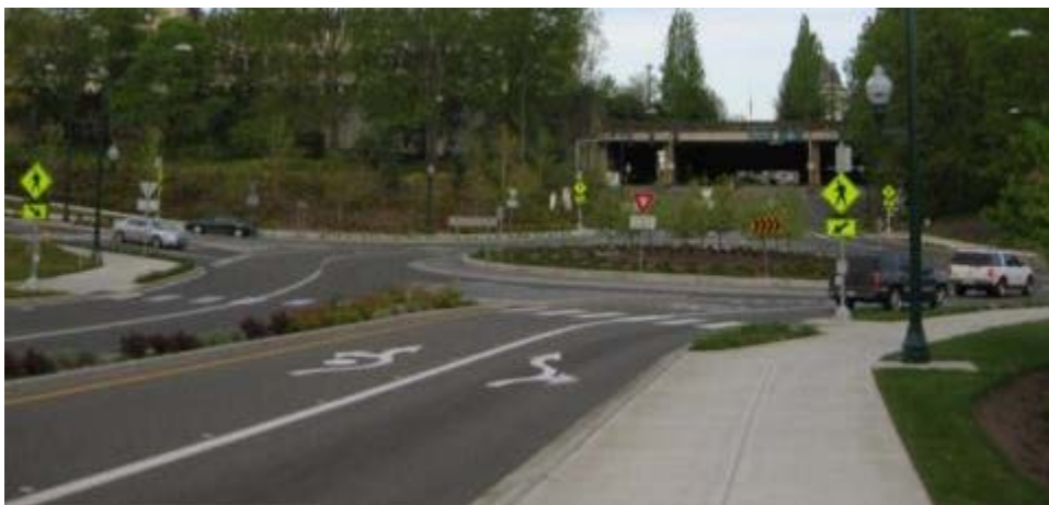
Figure 20. Photo. 14th Ave SE, east leg two-lane entry, two-lane exit, Olympia WA.
