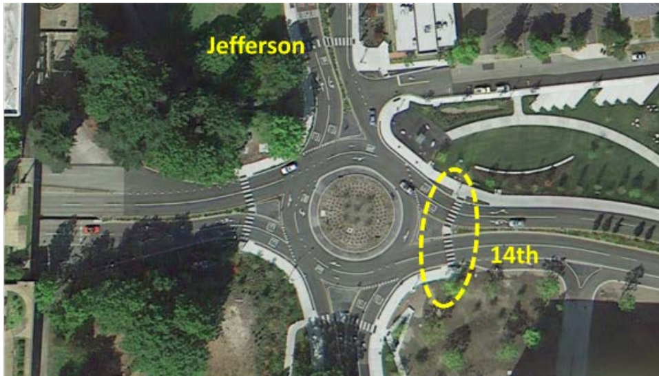
Figure 18. Photo. Aerial view of 14th and Jefferson roundabout in Olympia, WA.
