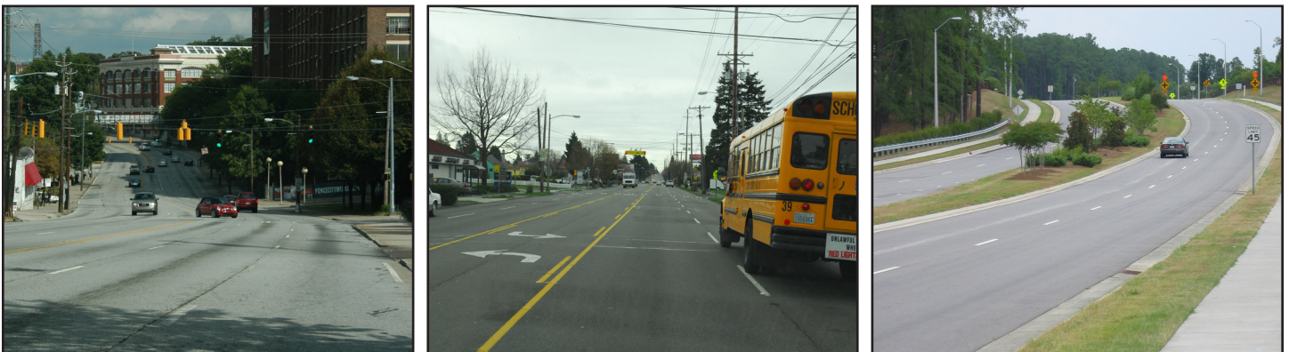
Exhibit 4: These photos illustrate (left) undivided roadway; (center) two-way left-turn lane; (right) raised median. (Source: VHB)
