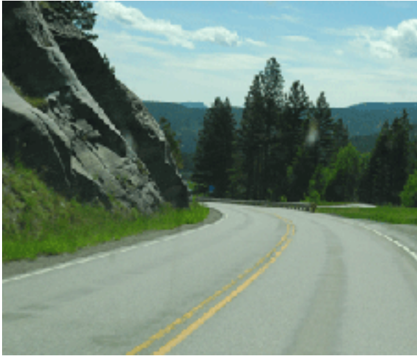
Horizontal curve near MP 107. An example of one of the many horizontal curves in the study area, the curve has limited sight distance, a pull-out located within the curve, and lacks signage.
