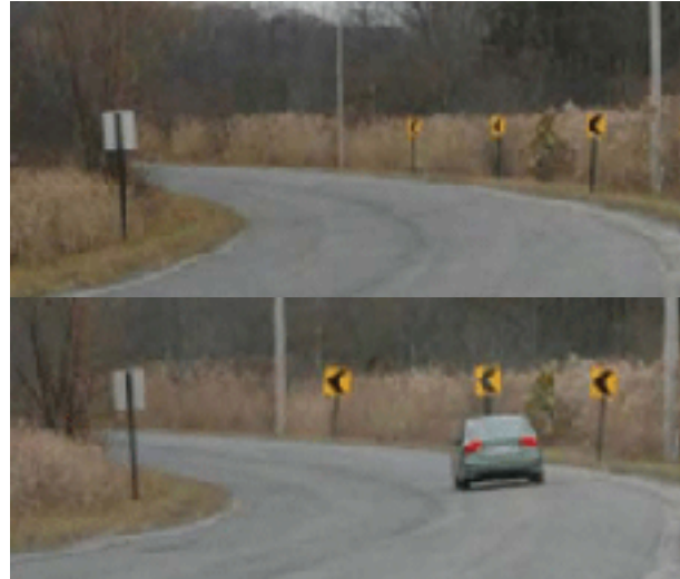
The upper photo is typical chevron size and placement. The lower photo demonstrates use of increasing chevrons, which include a slightly modified placement and placement so that they increase in size through the curve. (Source: Rensselaer Polytechnic Institute)
