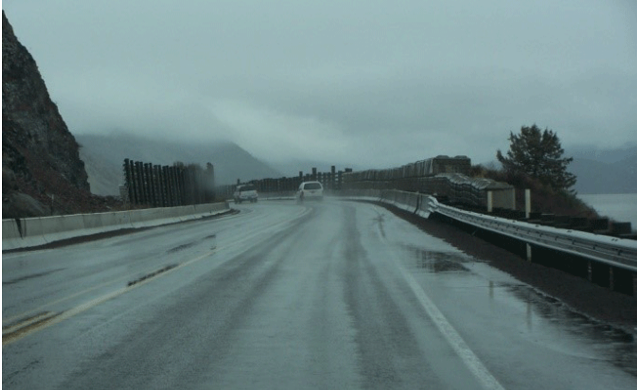
Figure 18: Sight distance is limited on horizontal curves with barriers.
