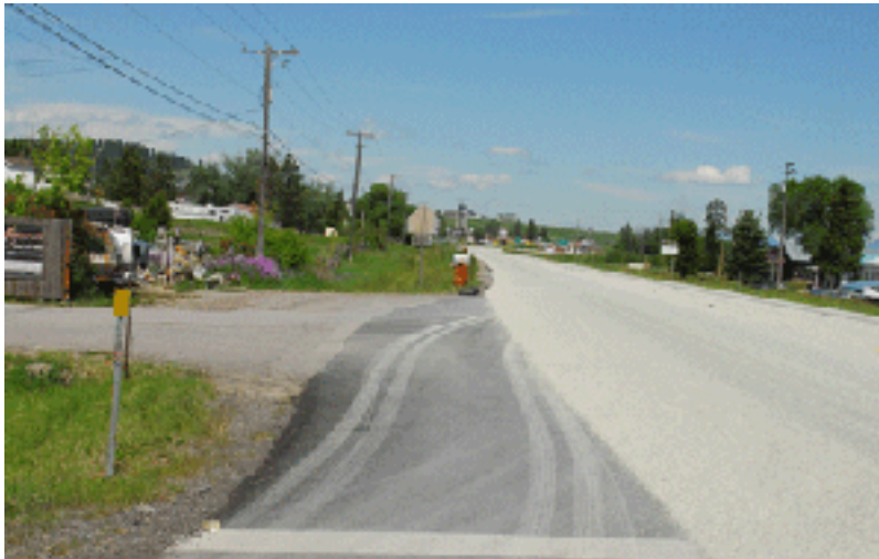
Eastbound view from intersection of US Highway 2 and Batavia Lane. Gas station access is to the left. Vehicles pull into the gas station to drop their kids off for school, requiring the students to cross Batavia to access the school. Vehicles park along the front of the intersection, potentially obstructing the view of students crossing Batavia in the crosswalk.
