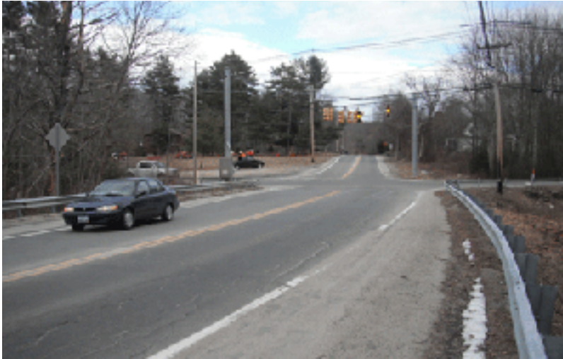
Conspicuity of Stop bar on eastbound approach is poor and loose debris is present in the shoulder.
