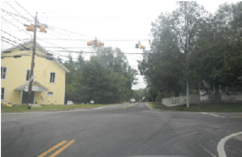
The flashing signal at the Sawmill Road intersection.
