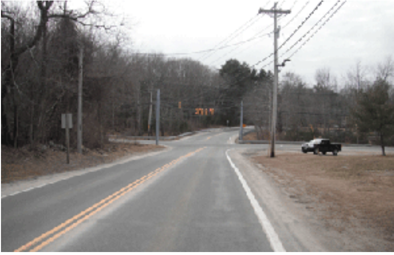
View of the intersection looking west, showing the horizontal curve west of the intersection (far-side). On the near-side of the intersection (east side) a utility pole and span wire pole are located in the clear zone.
