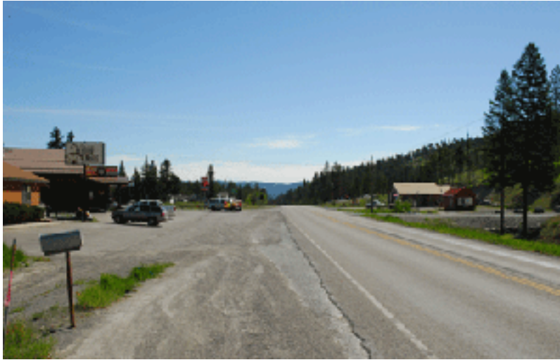
Eastbound view of intersection and parking/access locations just after horizontal curve. Motorists may not expect vehicles entering the roadway given the rural nature.
