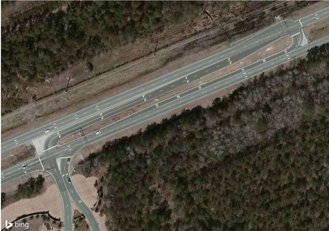
Exhibit 1-11. Three-legged RCUT intersection on US-17 at Brunswick Forest Parkway in Leland, NC. (2)
