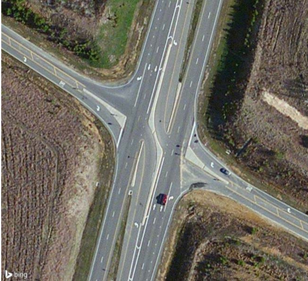
Exhibit 7-4. Stop-controlled RCUT intersection on US-1 near Southern Pines, NC. (2)
