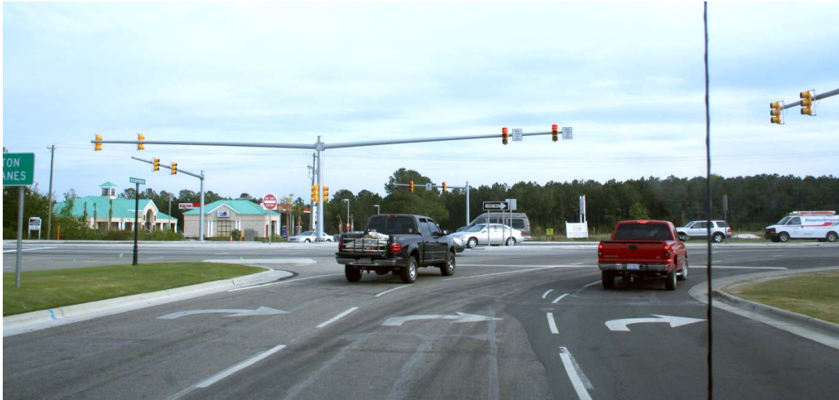
Exhibit 8-9. Signal pole locations on the minor street approaches of a RCUT intersection on US-17 in North Carolina. (3)
