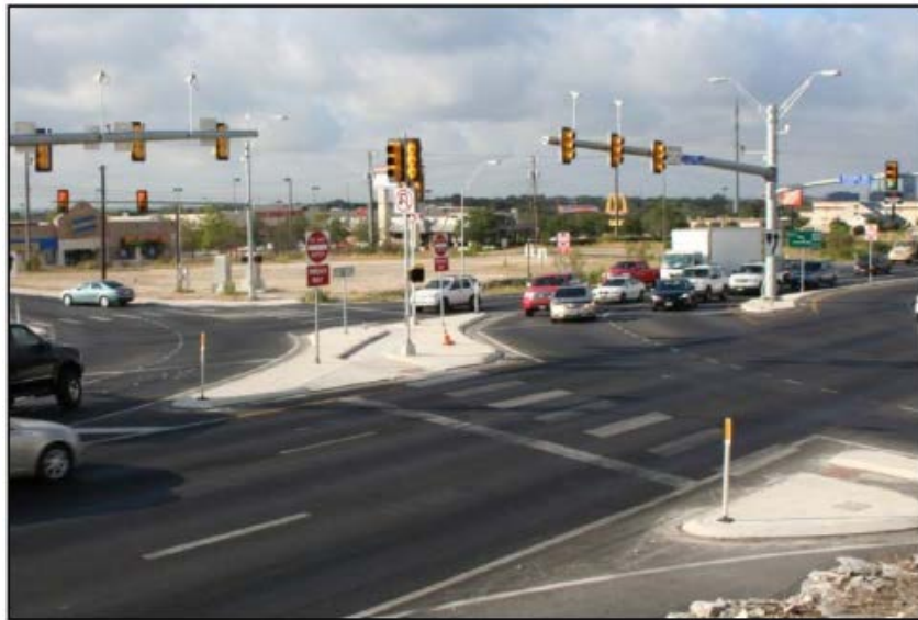
Exhibit 1-10. Signaled RCUT intersection in operation near San Antonio, TX showing a pedestrian “Z” crossing. (3)
