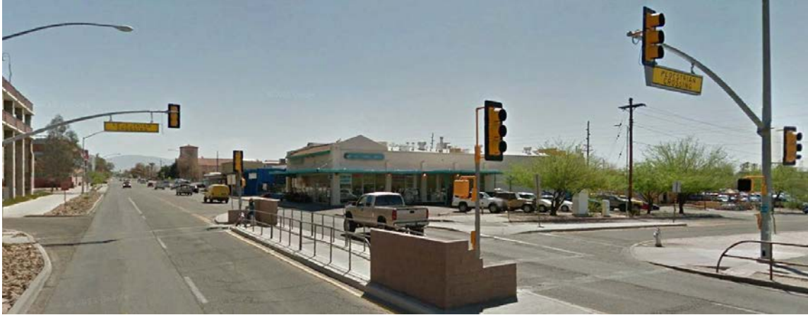
Exhibit 3-10. Two-stage channelized pedestrian crossing at conventional intersection. (25)
