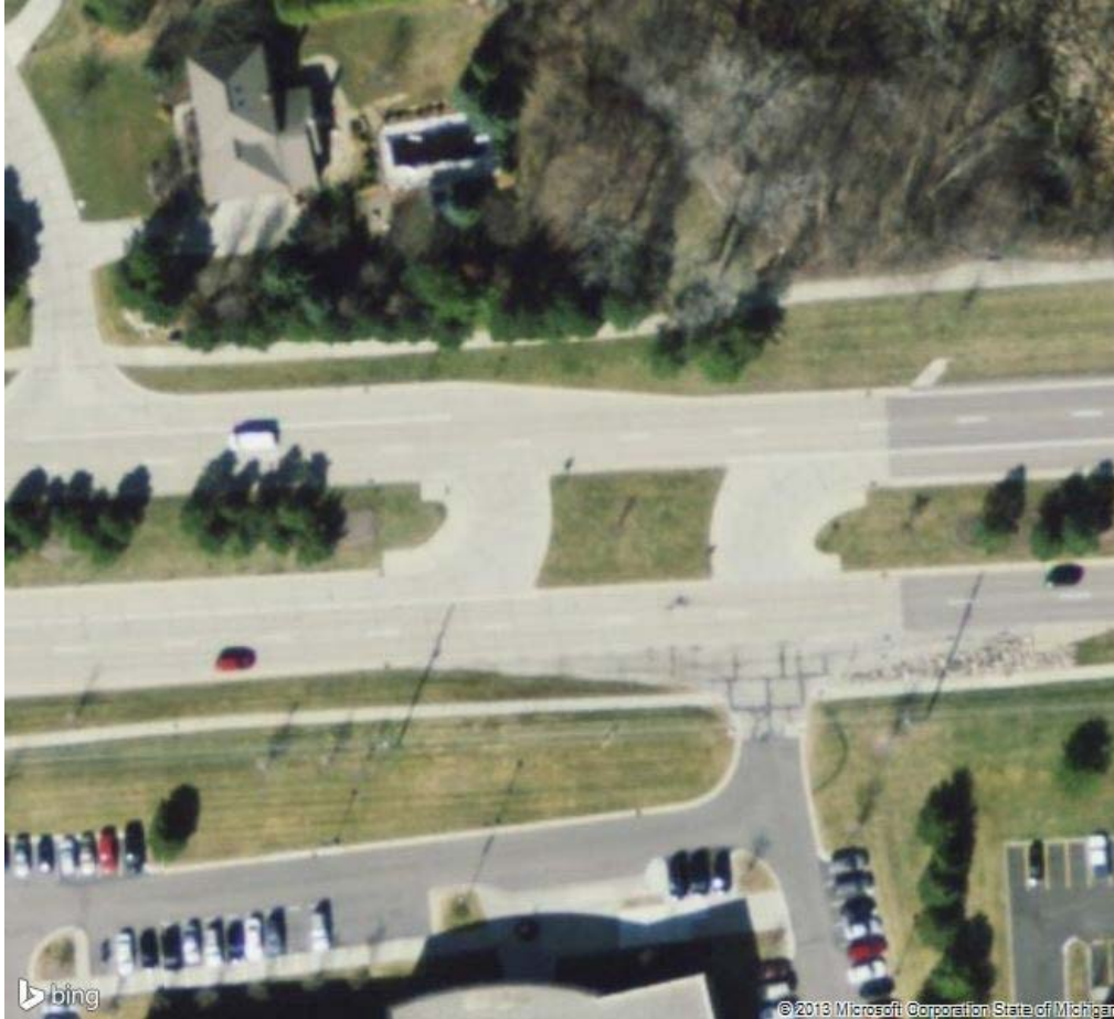
Exhibit 7-17. Other treatments used at U-turn crossovers on Twelve Mile Road in Farmington Hills, MI to accommodate large vehicles. (2)
