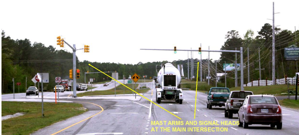
Exhibit 8-6. Signal pole locations at the main intersection of a RCUT intersection on US-17 in North Carolina. (3)
