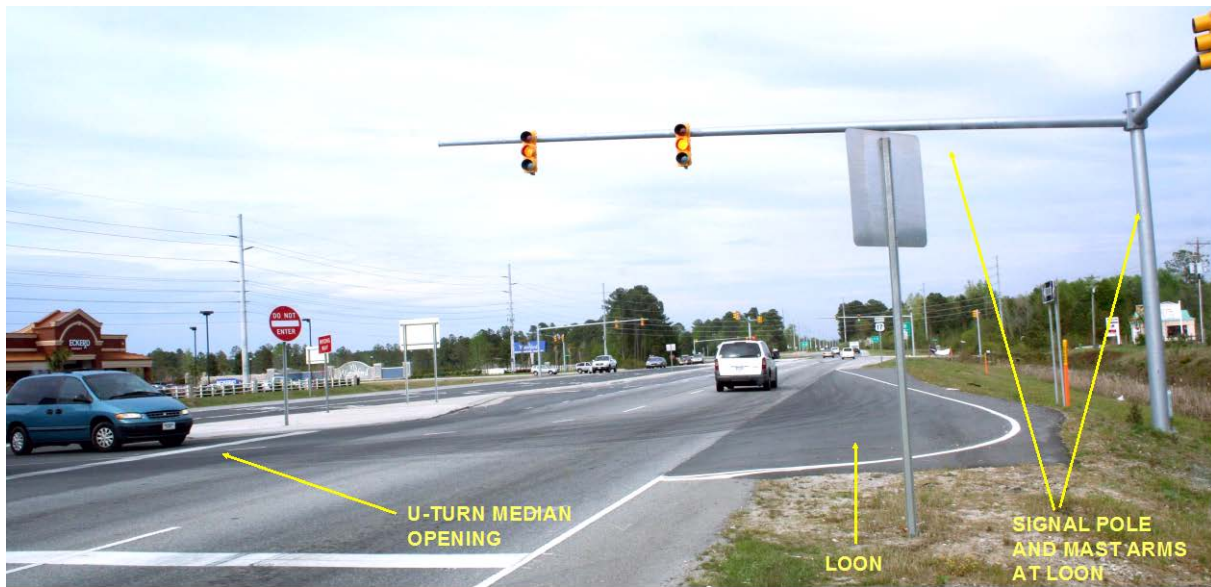
Exhibit 8-8. Signal pole locations at the U-turn crossover of a RCUT intersection on US-17 in North Carolina. (3)
