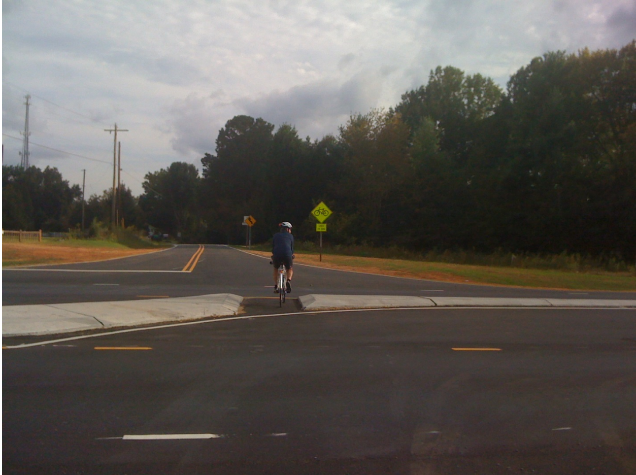
Exhibit 3-13. Curb cut design used in North Carolina to assist bicyclists crossing at a rural RCUT with stop sign. (27)
