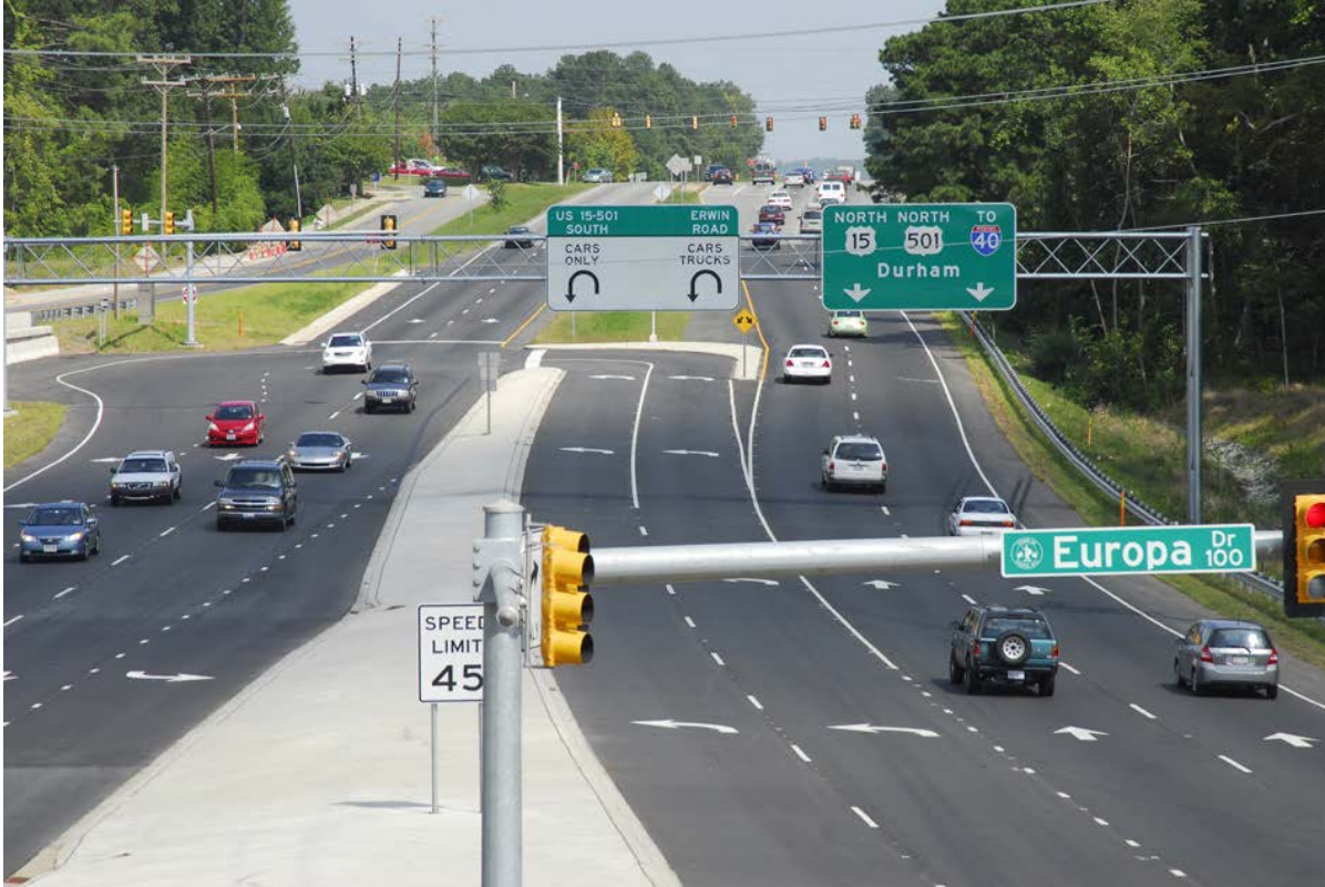
Exhibit 8-15. Overhead guide signs at the RCUT intersection on US-15/501 in Chapel Hill, NC. (27)
