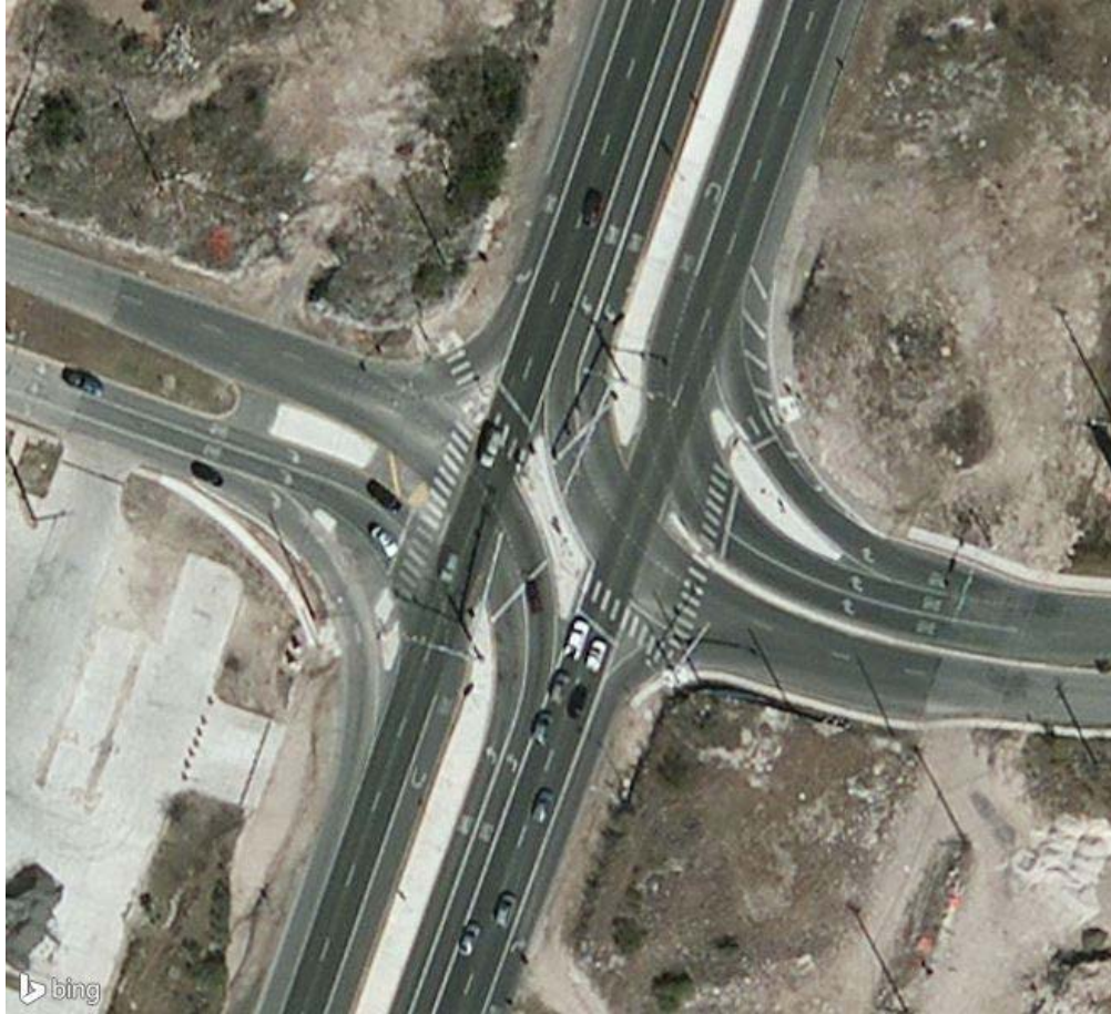
Exhibit 1-5. Signalized RCUT intersection on US-281 in San Antonio, TX with four-lane major street and four-lane minor street. (2)
