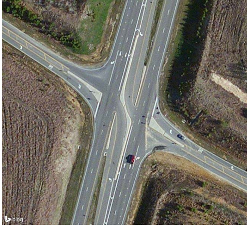
Exhibit 1-6. Stop-controlled RCUT intersection on US-1 near Southern Pines, NC. (2)
