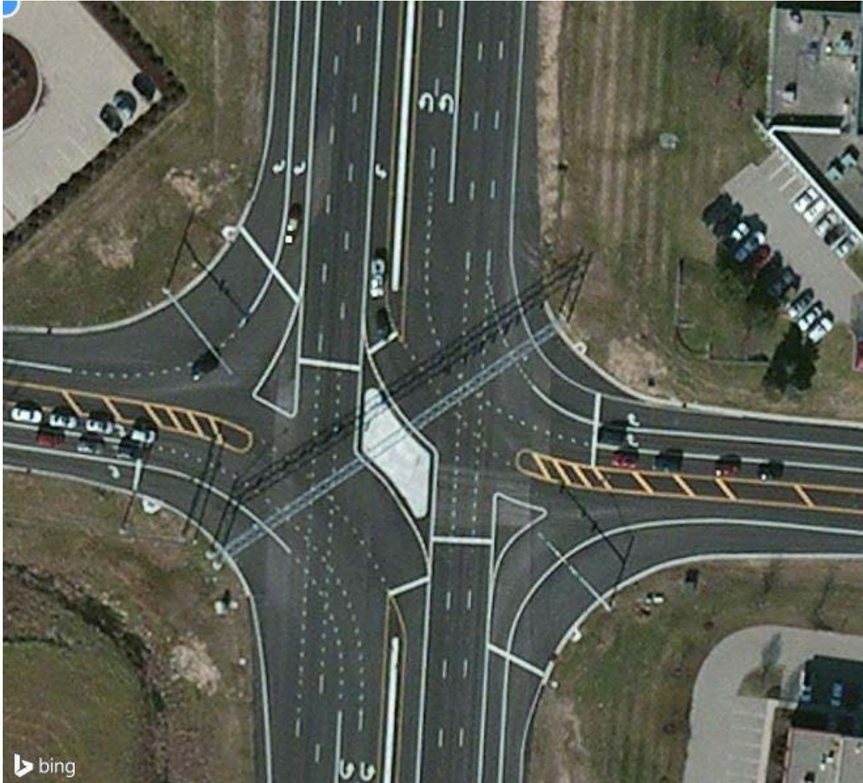
Exhibit 7-6. Signalized RCUT intersection on OH-4 outside Hamilton, OH with six-lane major highway and four-lane minor road. (2)
