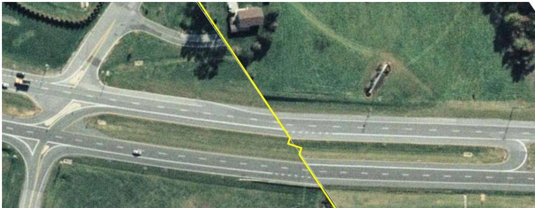
Exhibit 1-7. Merge-controlled RCUT intersection on US-15 in Emmitsburg, MD. (3)
