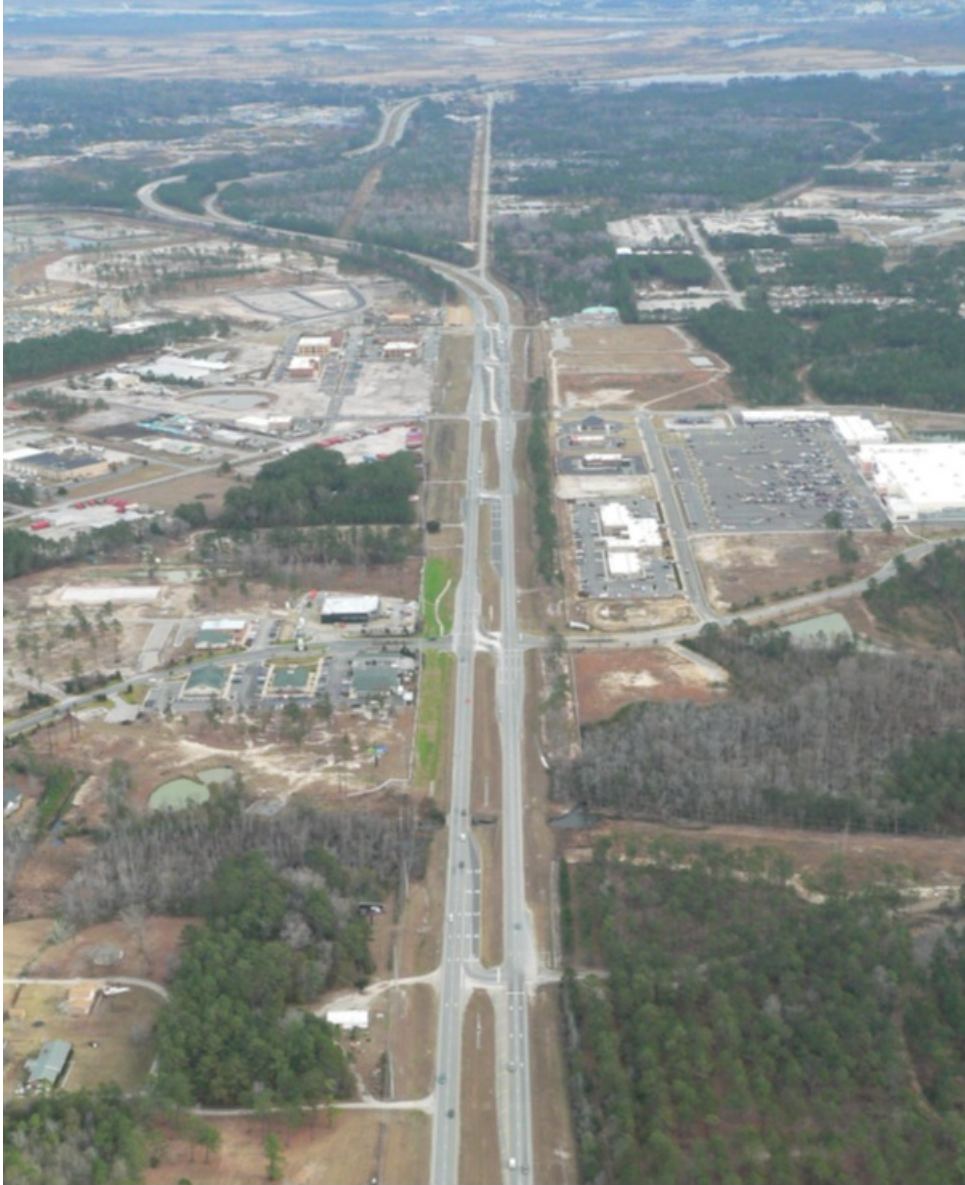
Exhibit 1-12. RCUT corridor on US-17 in Leland, NC. (4)
