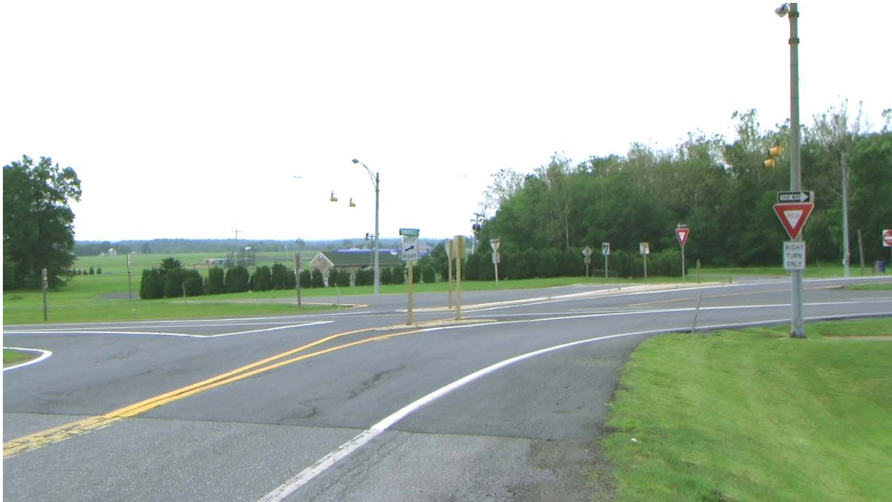
Exhibit 8-17. Signing at a merge-controlled RCUT intersection in Emmitsburg, Maryland. (3)
