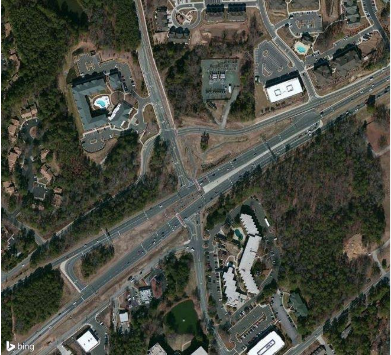
Exhibit 1-8. RCUT intersection on US-15/501 in Chapel Hill, NC with no left-turn crossovers. (2)
