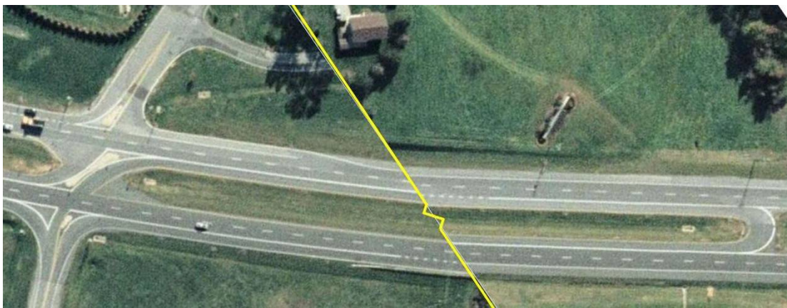
Exhibit 7-5. Merge-controlled RCUT intersection on US-15 in Emmitsburg, MD. (3)
