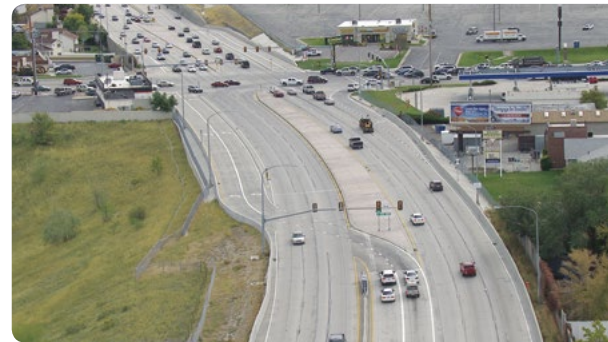
Left Turn Crossover at Bangerter Highway and 3500 South Source: DLT Case Study Video FHWA-SA-14-059
