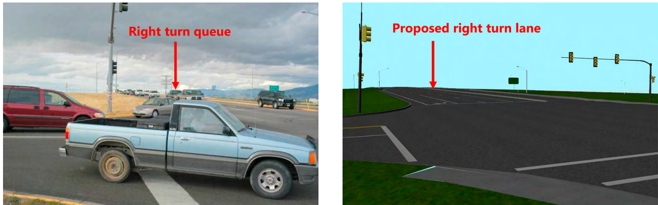
Figure 18: Southbound right turn at the intersection of Jackrabbit Lane /Amsterdam Road – Existing (L) and Modeled (R) Views Significant right-turn traffic volume obstructs view of approaching through vehicles
