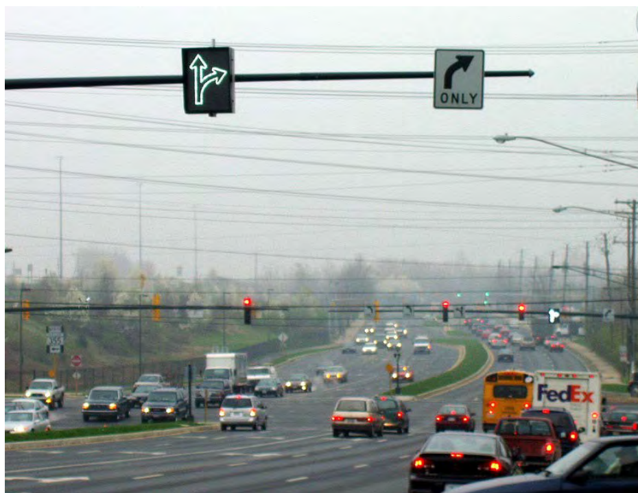
Exhibit 11-31. Example use of variable lane use sign to add a second right-turn lane along a corridor during certain times of day.
