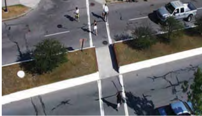
Exhibit 8-5. This refuge island enables two-stage pedestrian crossings.
