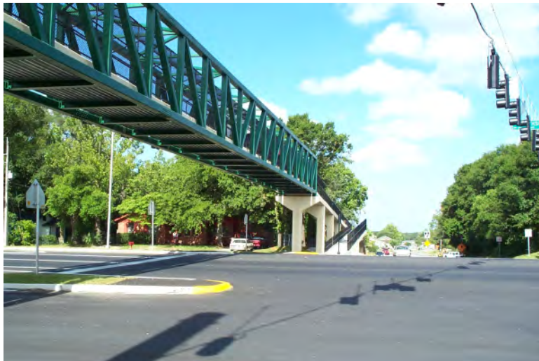
Exhibit 4-15. A pedestrian grade separation treatment restricts sight distance of the traffic signal as motorists approach the intersection.
