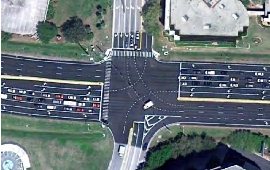
Exhibit 4-9. The photo shows how double and triple left-turn lanes can be used to accommodate high-priority movements. Source: Google 2012
