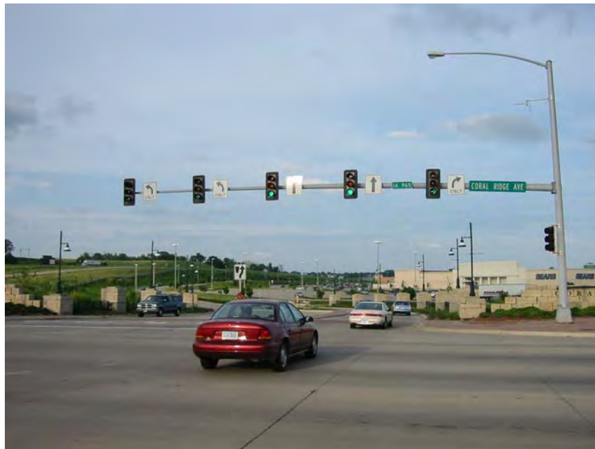
Exhibit 10-7. Lane-aligned signal heads.
