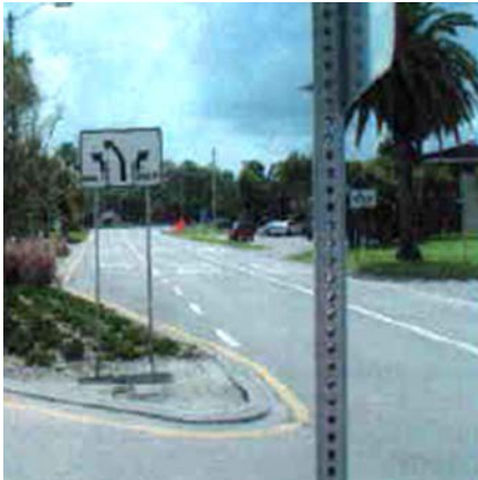
EB median nose at plaza just east of 41st St. SW (before).
