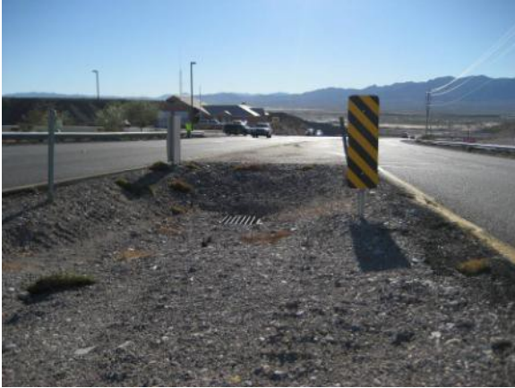
Nontraversable median drains.
