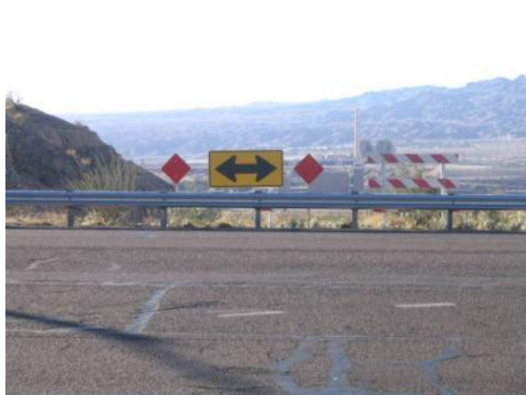
Enhanced T-intersection signing.
