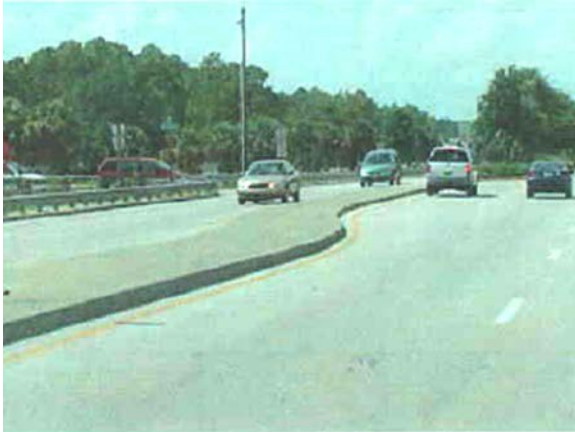
SB left-turn lane to 25 th Ave. SW (before).
