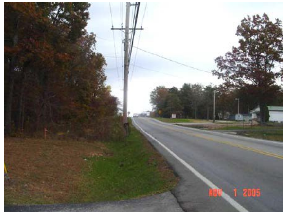
Vertical alignment looking north at L.M. 18.50 to L.M. 18.70.
