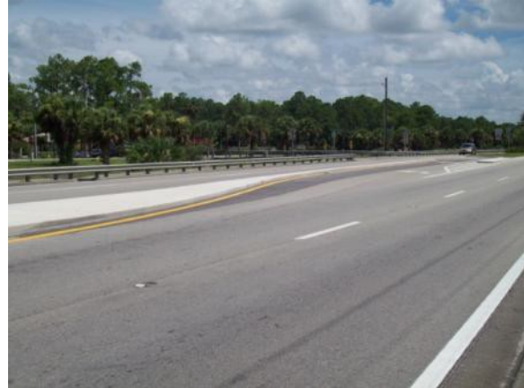
SB left-turn lane to 25 th Ave. SW (after). SB left only; no WB left.
