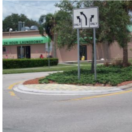
EB median nose at plaza just east of 41st St. SW (after). Nose cut back.
