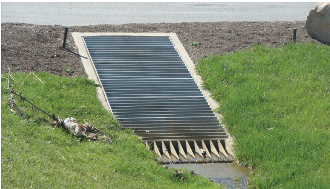
Grated inlet flush with ground over a culvert end.
