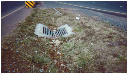
V-shaped grate in median.
