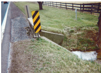
Rigid headwall delineated with Type 3 Object Marker.
