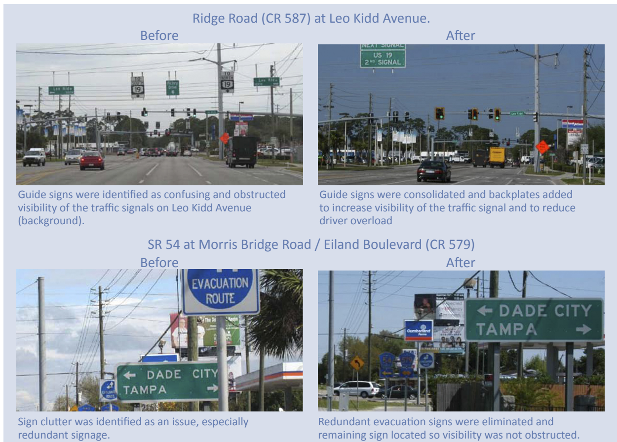
Figure 5. Examples of Issues Identified during Pasco County RSAs.
