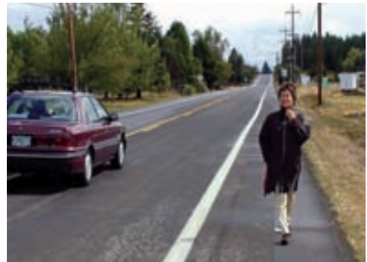
Paved shoulders offer pedestrians on rural roadways a safer place to walk.
