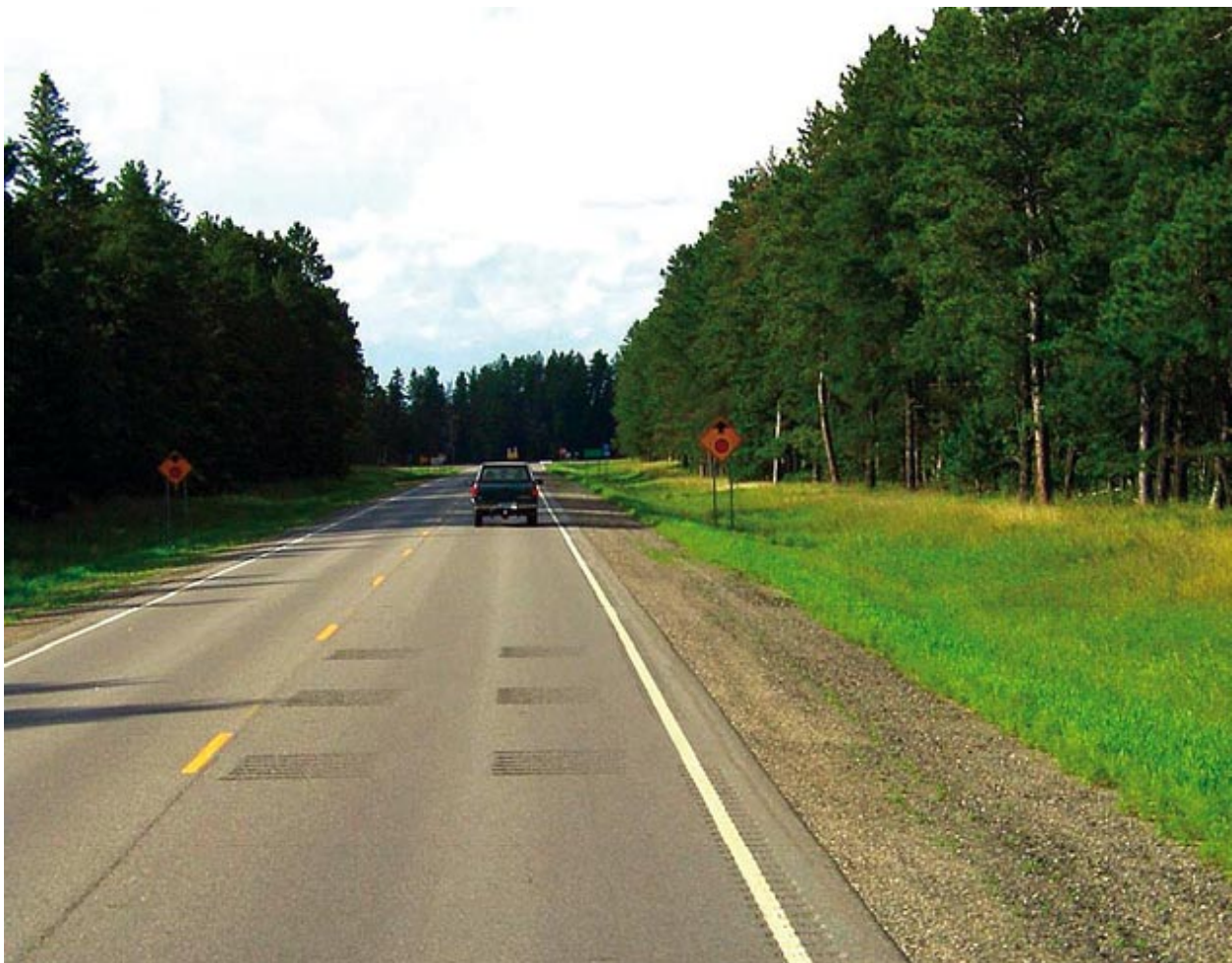
Figure 41. Transverse rumble strip (31).
