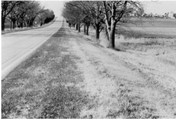
Typical Roadway with Roadside Hazard Rating Equal to 5.
