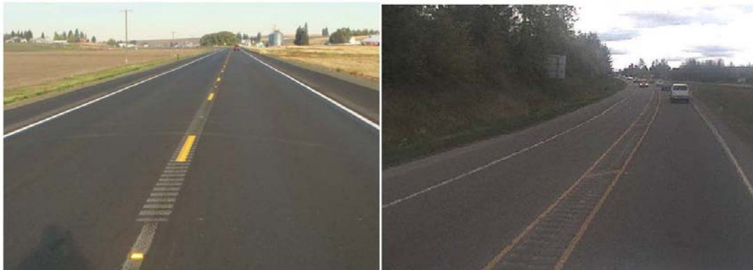
Figure 20. Centerline rumble strips (milled) (23).
