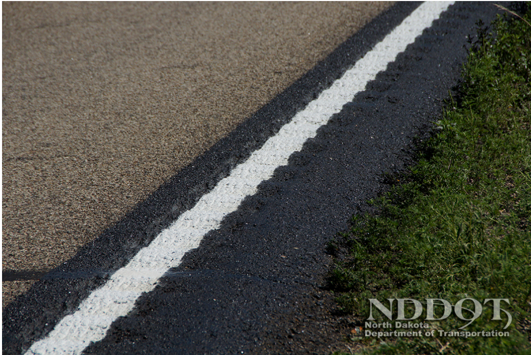
Figure 10. Right shoulder milled or rolled on/under edgeline (22).
