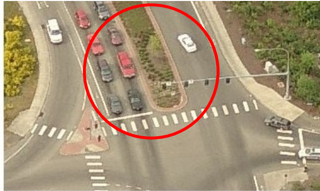
Raised With Curb
