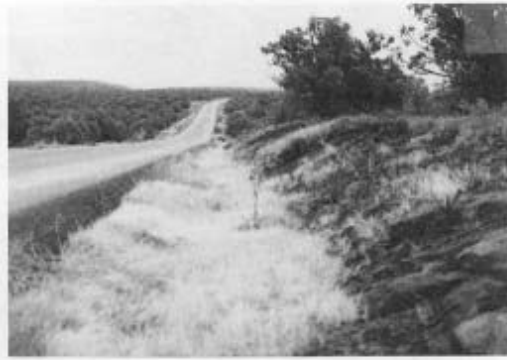
Rural roadside hazard rating of 3.
