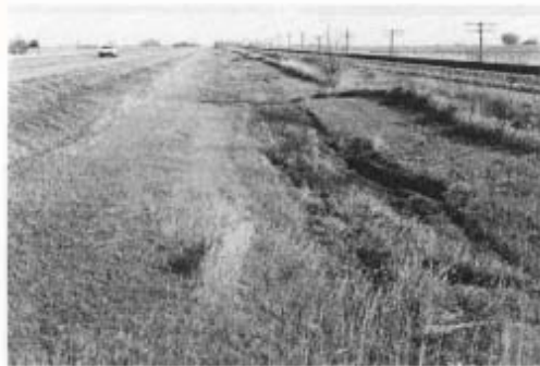
Rural roadside hazard rating of 2.
