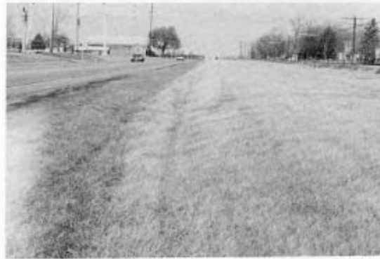
Rural roadside hazard rating of 1.
