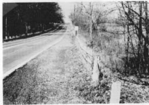
Rural roadside hazard rating of 5.
