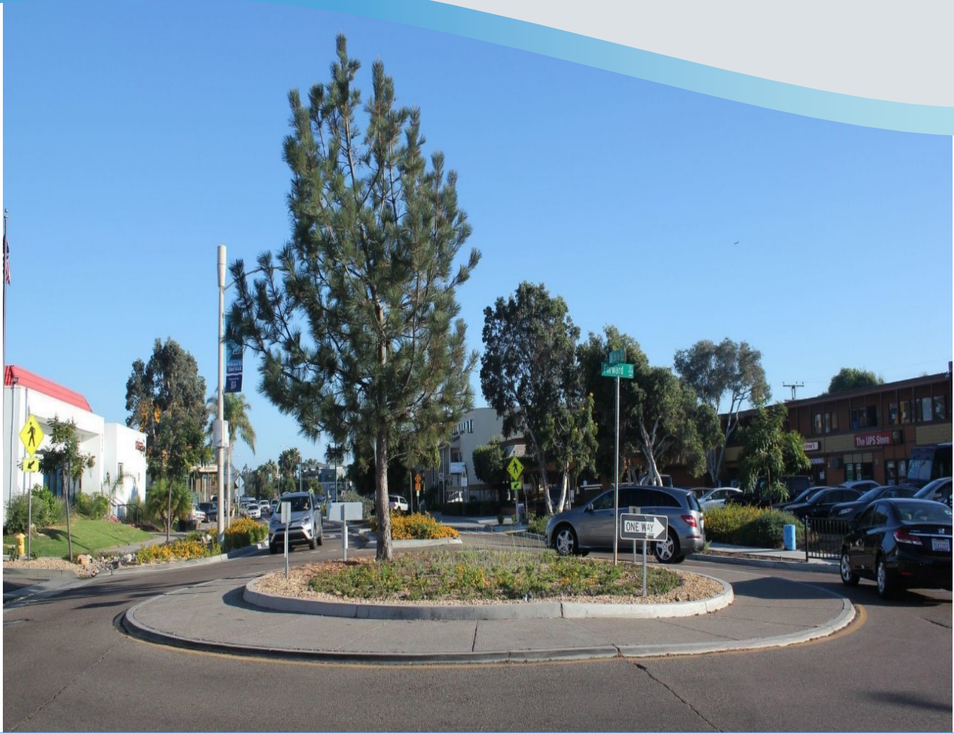
Figure 3. Graphic. A roundabout installation in San Diego.
