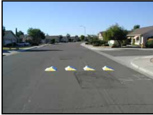
Figure 4. 3-D Markings on 85 th Lane in Peoria
