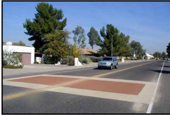
Figure 7. Tyregrip™ Installation on Coral Gables Drive in Phoenix
