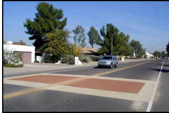
Tyregrip™ installation on Coral Gables Drive in Phoenix
