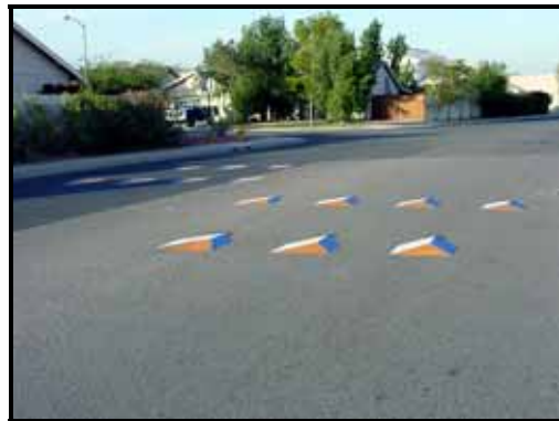
Figure 6. 3-D Markings on Pavement Between Speed Tables on 84 th Avenue in Peoria
