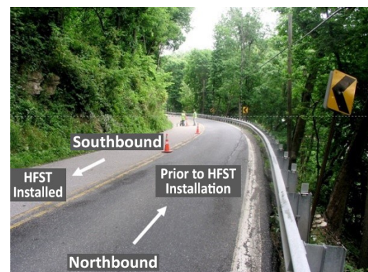
Figure 2: HFST Pilot Project. Source: PennDOT
