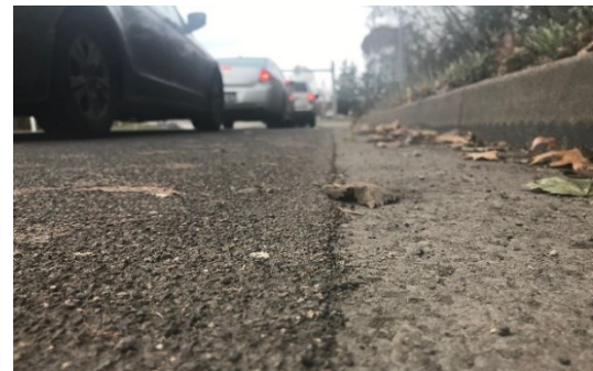
Figure 9: Boundary between HFST and Pavement Surface. Source: PennDOT
