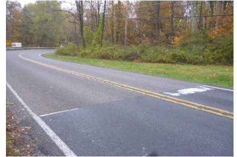
Figure 11: Typical HFST Application on Rural Two-Lane Road. Source: PennDOT
