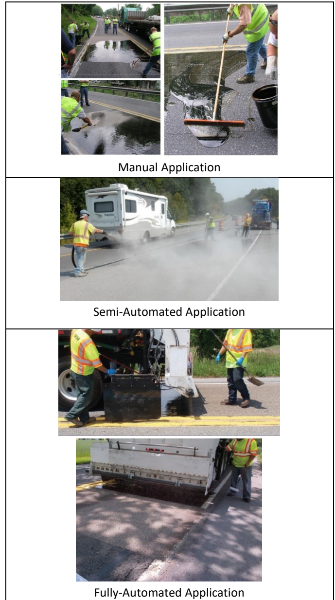
Figure 7: Three Primary Application Methods. Source: PennDOT
