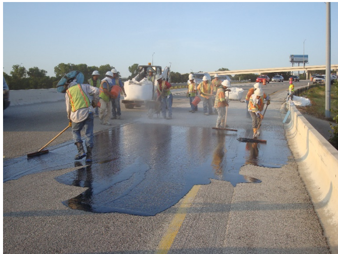
Figure 65. Photograph. Manual application of HFST to bridge deck.
