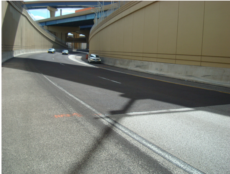
Figure 38. Photo. Example of aggregate shedding and accumulation along lane edge and on paved shoulder.
