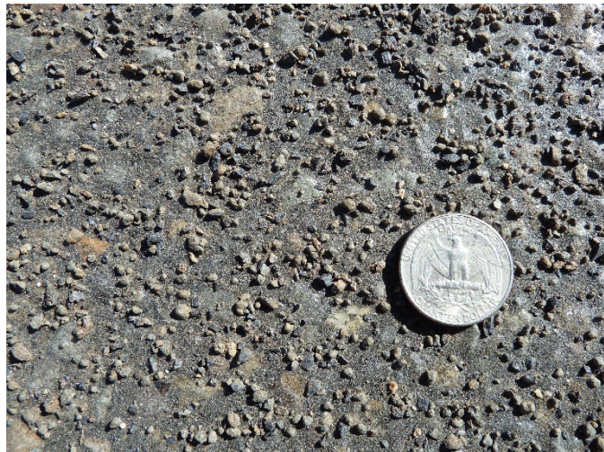
Figure 47. Photograph. HFST with inadequate aggregate coverage due to delayed aggregate application.
