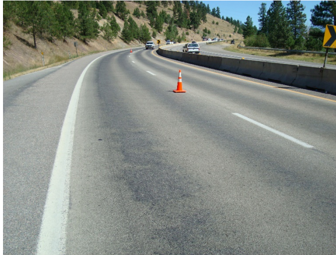
Figure 42. Photo. Example of HFST worn off in the wheelpaths.
