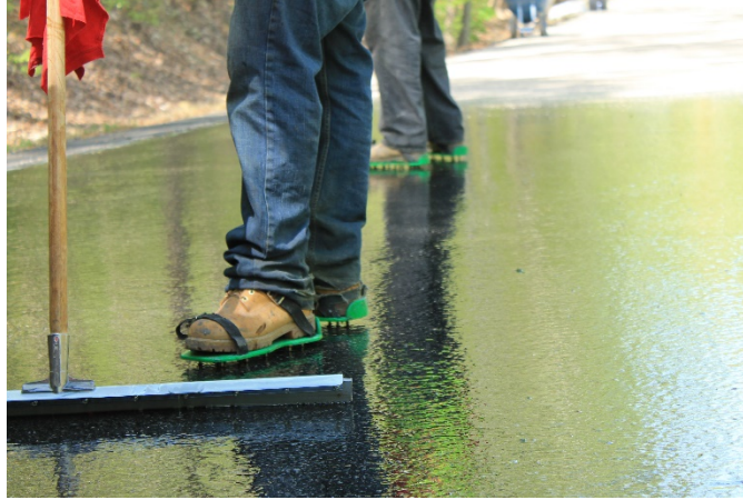
Figure 27. Photo. Example of spiked shoes worn by squeegee operator.
