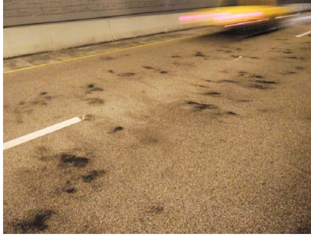
Figure 45. Photograph. Example of soft areas in resin binder shortly after construction (FDOT 2021).
