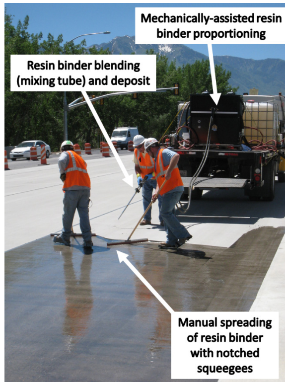
Figure 13. Photograph. Example of mechanically-assisted manual resin binder application.
