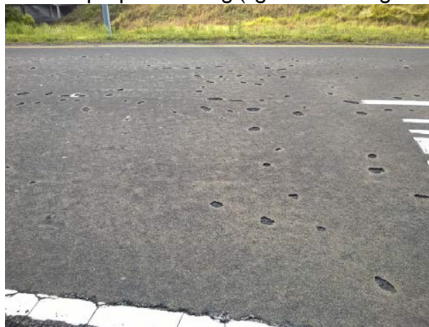
Figure 44. Photograph. Example of localized failures due to poor binder mixing (FDOT 2021).
