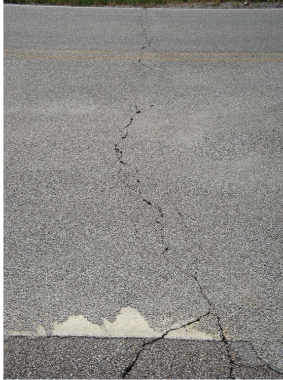
Figure 51. Photograph. Example of cracking in underlying pavement reflecting through HFST.
