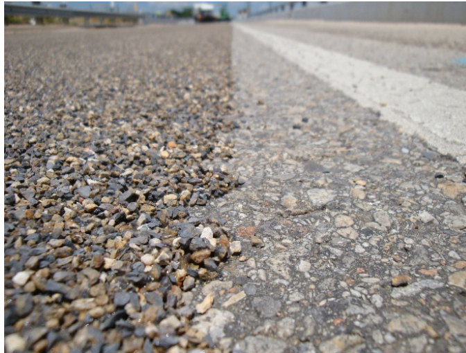
Figure 18. Photograph. HFST placed over a conventional asphalt pavement surface (Merritt et al. 2020a).
