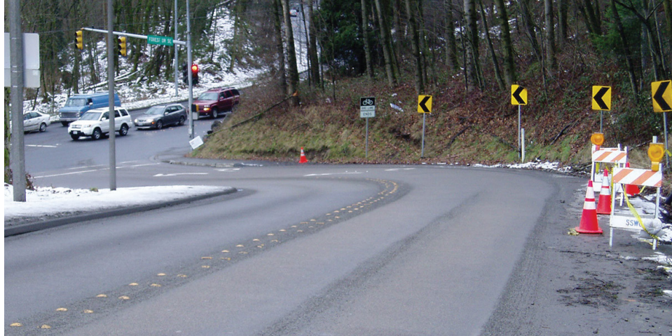
Figure 57. Photograph. HFST application for steep grade at intersection approach (FHWA 2016).
