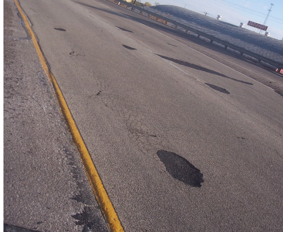
Figure 43. Photo. Example of failure of underlying pavement leading to isolated failures (potholes) of HFST.
