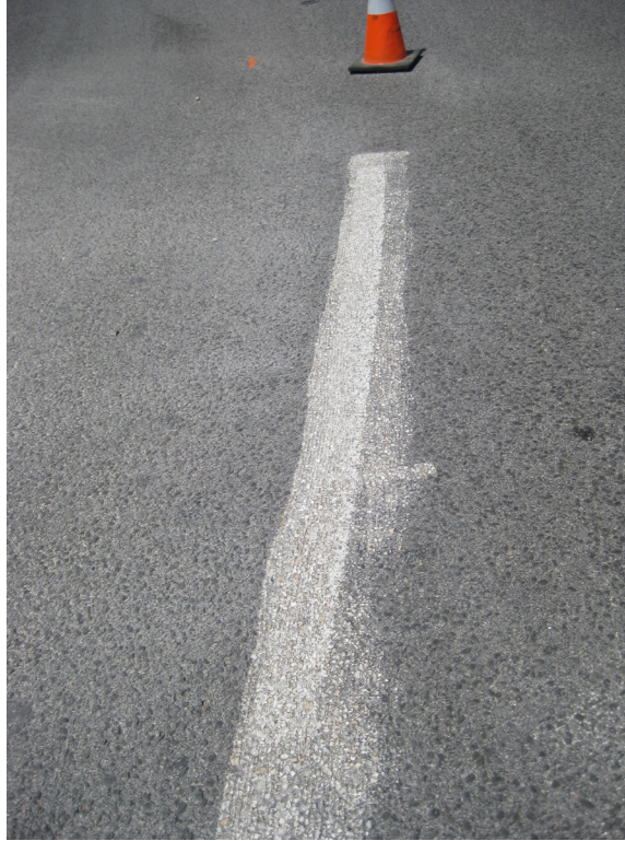
Figure 23. Photo. Example of pavement striping removal using milling which has not damaged the underlying pavement.
