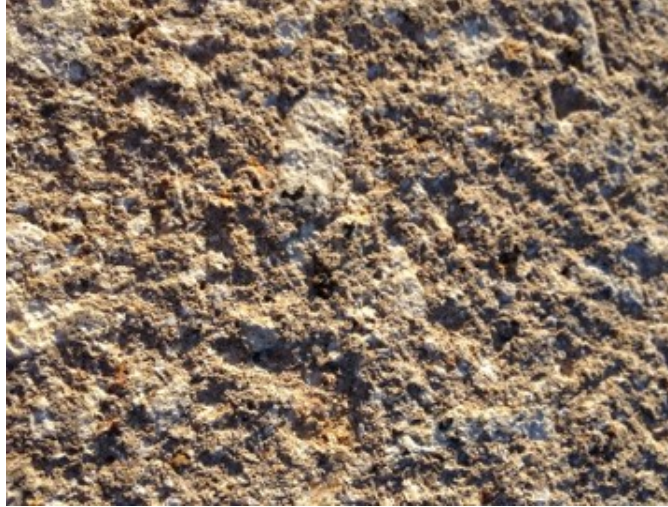
Figure 22. Photo. Shotblast concrete surface with CSP = 5.
