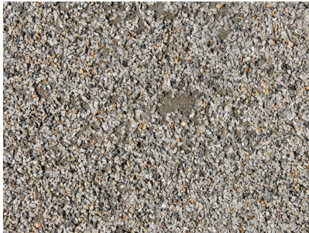
Figure 46. Photograph. Example exposure of underlying pavement due to inadequate resin binder thickness.
