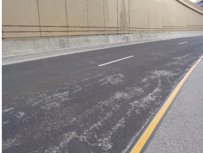
Figure 52. Photograph. Example of aggregate loss under traffic wear.
