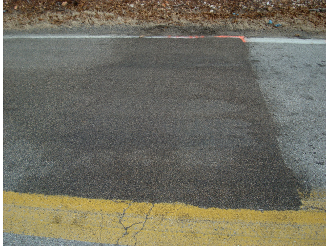
Figure 36. Photo. Example of discoloration indicating uncured resin binder.
