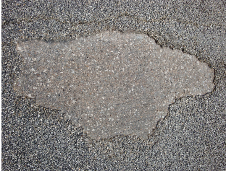
Figure 39. Photo. Example of delamination of HFST from underlying pavement surface.
