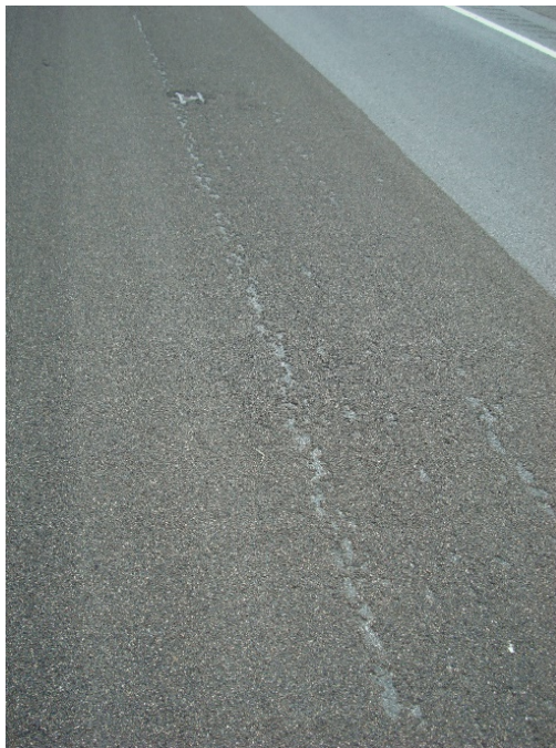
Figure 36. Photo. Example of discoloration indicating uncured resin binder.
