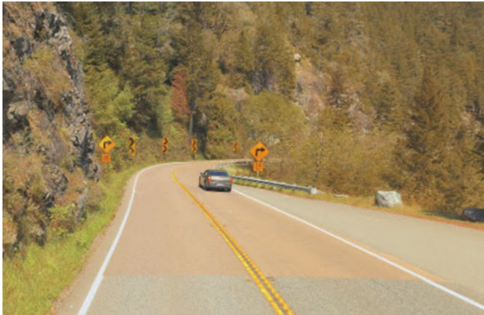
Figure 54. Photograph. Example of HFST as an alternative to curve realignment (FHWA 2015).
