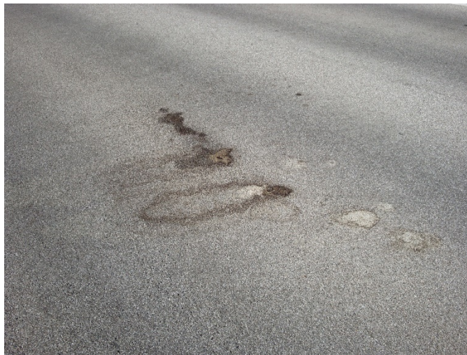
Figure 41. Photo. Example of HFST discoloration likely caused by moisture.
