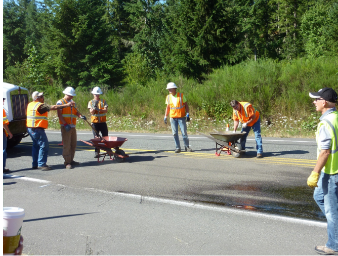
Figure 30. Photo. Example of manual application of HFST aggregate.
