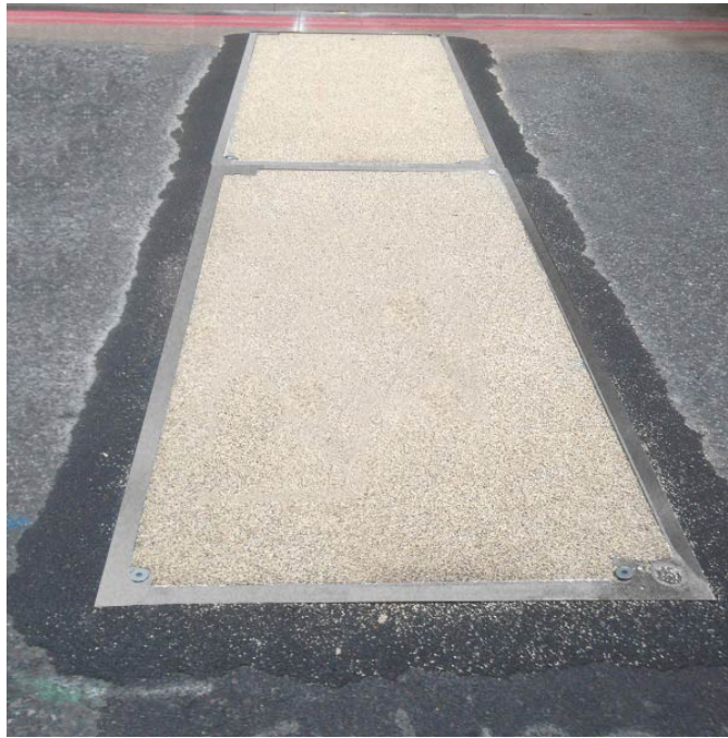
Figure 66. Photograph. HFST with calcined bauxite on steel trench plates (Heaton Manufacturing n.d.).
