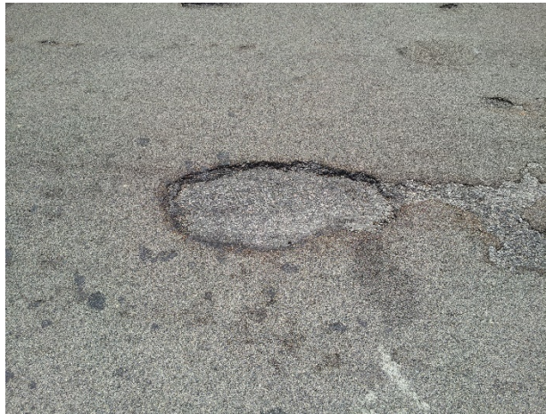
Figure 49. Photograph. Example failure of underlying pavement (delamination of surface layer) resulting in failure of HFST.
