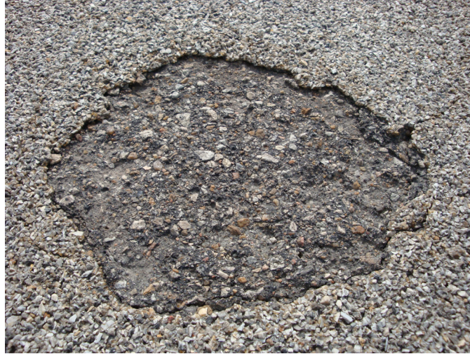
Figure 48. Photo. Example of an area of HFST delamination from the underlying pavement surface.
