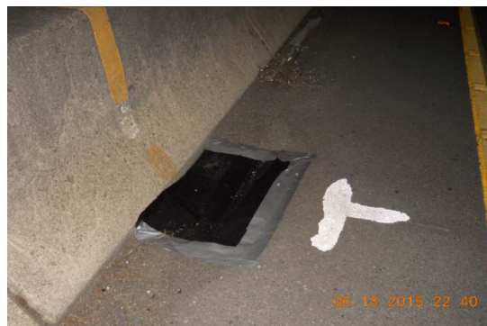
Figure 24. Photo. Example of masking of drainage structures near HFST application.
