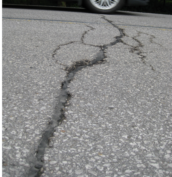
Figure 19. Photo. Example of bituminous crack sealant in asphalt pavement recessed from the top surface of the pavement.
