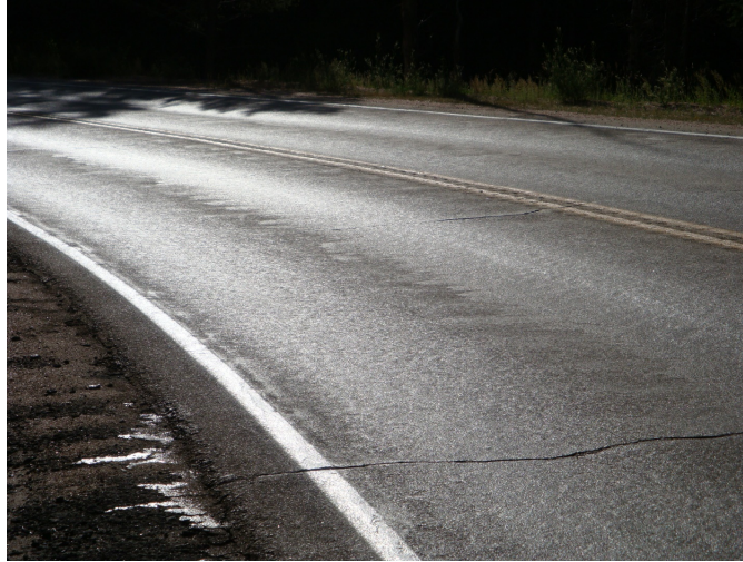
Figure 40. Photo. Example of polished HFST surface in wheelpaths.
