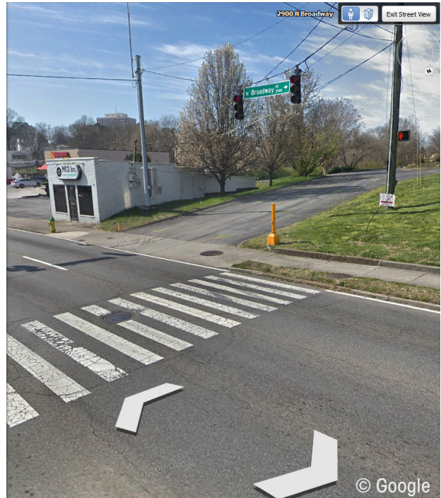
Figure 3. Photograph. Google Streetview image of marked crosswalk at a signalized intersection during RSA corridor review.
