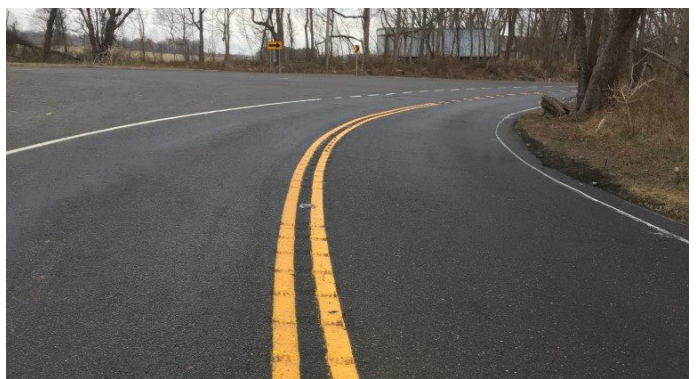
Figure 2. Center line rumble stripes in Mercer County reduce head-on crashes. Source: George Fallat, Mercer County, New Jersey.
