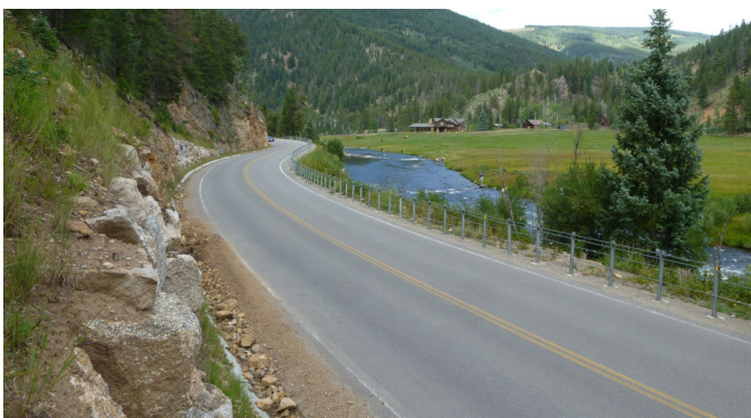
Figure 3. A high-tension cable barrier preserves views of the landscape while shielding vehicles from a steep drop-off. Source: FHWA.
