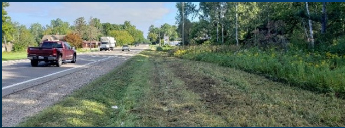
Figure 5. Roadside tree removal is followed up with mowing to reduce the chances of fixed-object crashes. Source: Destain Gingell, Lapeer CRC.
