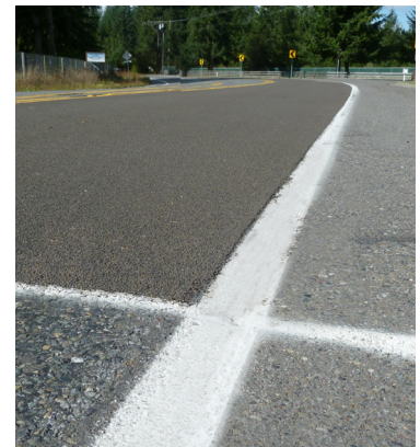
Figure 4. HFST at a Thurston demonstration site. Source: FHWA.
