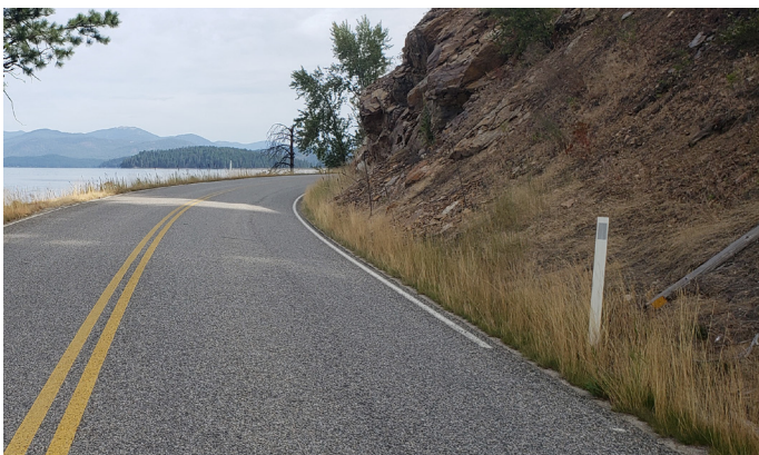
Figure 1. Edge lines and delineators improve visibility on horizontal curves. Source: Matt Mulder, Bonner County, Idaho.
