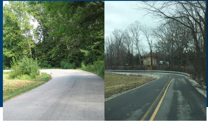
Figure 6. Before and after curve safety improvements that include centerline marking, guardrail, and cutting back vegetation to improve sight distance. Source: Indiana LTAP.
