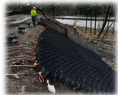
Below: Placement of topsoil on reinforced soil slope wall
