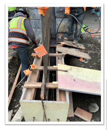
North Wing Wall Foundation Concrete Pour in West Portal
