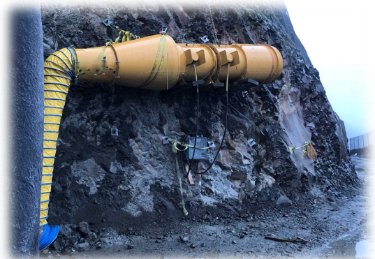
West portal ventilation system installed
