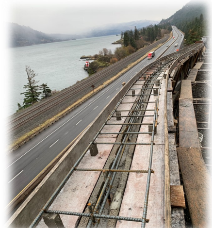
Left & Right: Rebar and form work at East retaining wall railing cap
