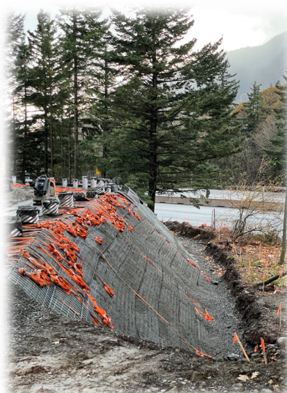
Construction of reinforced soil slope
