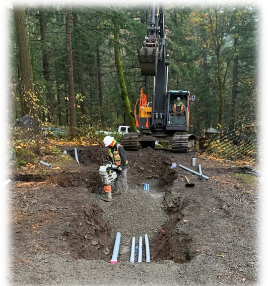
Installation of underground utilities
