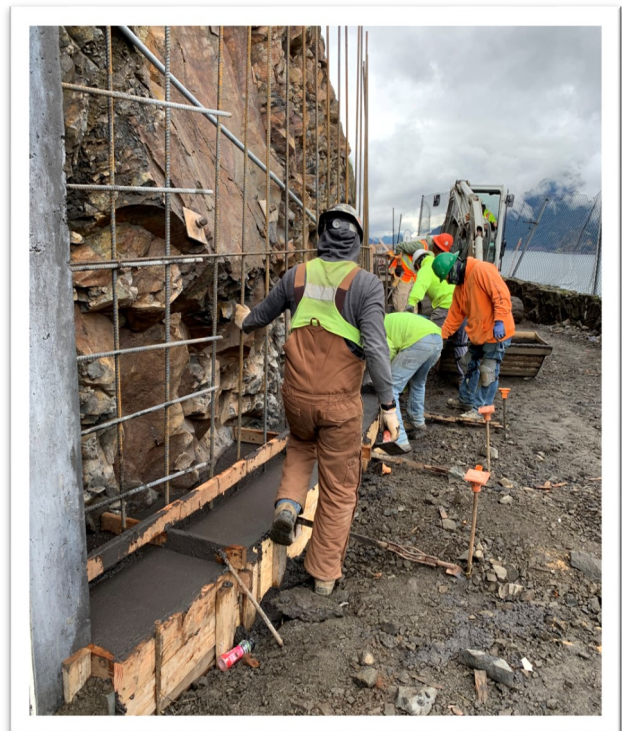
South Wing Wall Foundation Concrete Pour in West Tunnel Portal
