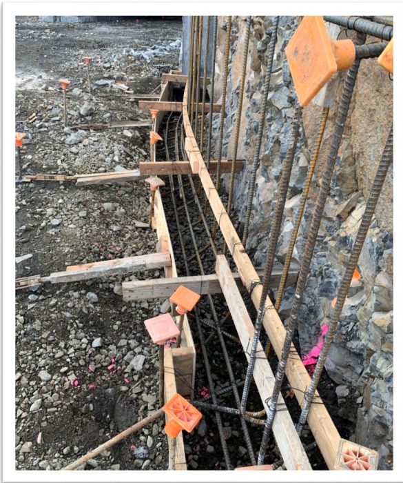
Concrete Form and Rebar ~ South Wing Wall in West Tunnel Portal
