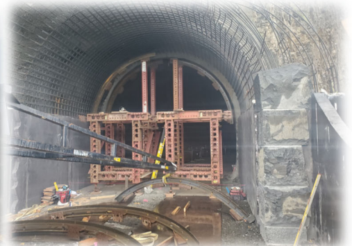
Below: Forming arch at East Portal
