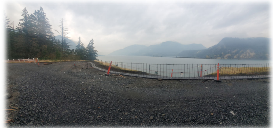
Below: Footing for wall on the West side
