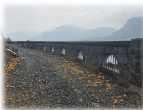
Below: Stone facing progress on East Bench
