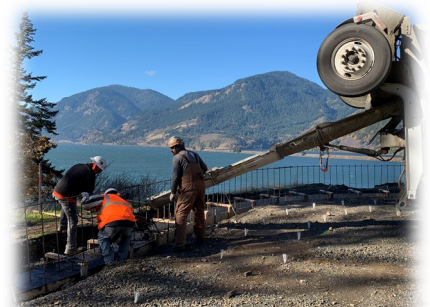
Below right: Concrete pouring retaining wall foundation at West bench
