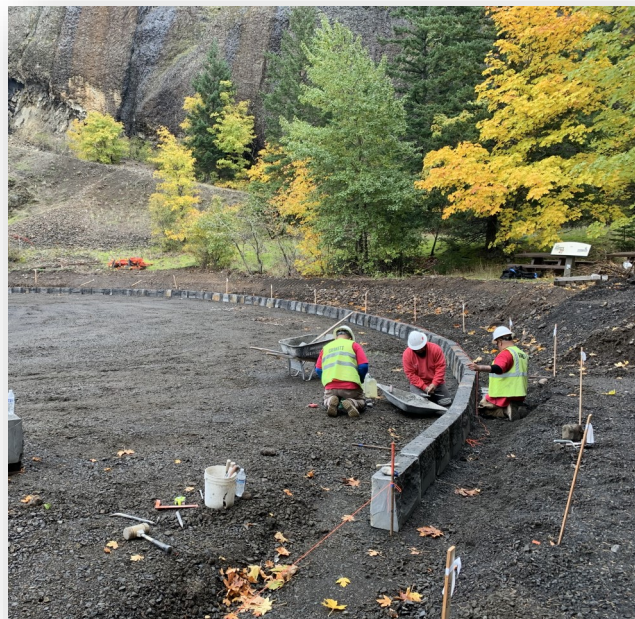
Curb Stone Installation at West Parking Lot
