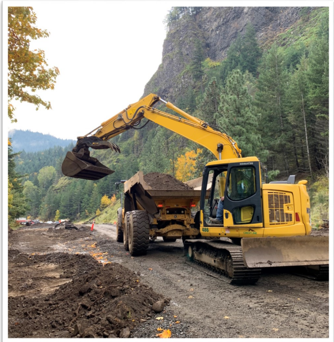
Storm Water Drainage Excavation In East Meadow
