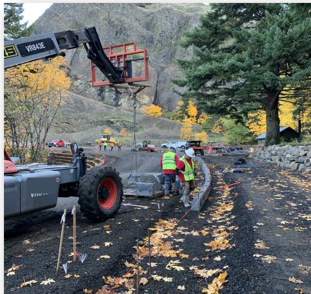
Curb Stone Installation at West Parking Lot
