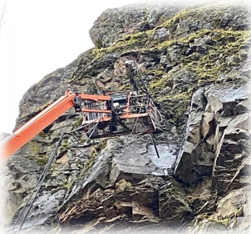
Left: Drilling holes for Rock Bolts
