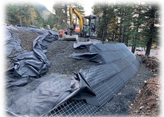
Below left and right: Building reinforced soil slope
