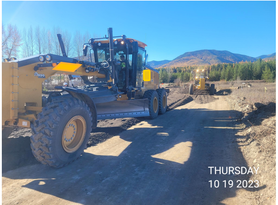
Placing Millings on Glacier Drive
