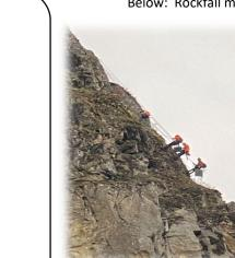
Below: Rockfall mitigation and hanging wire mesh at Stepped Cut
