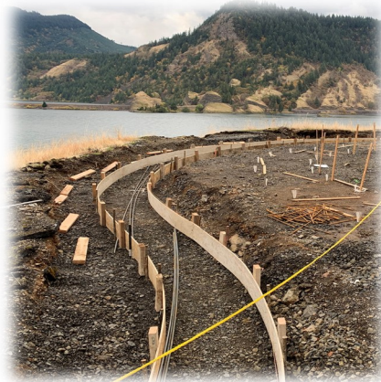
Below: Foundation forming and rebar at West Bench
