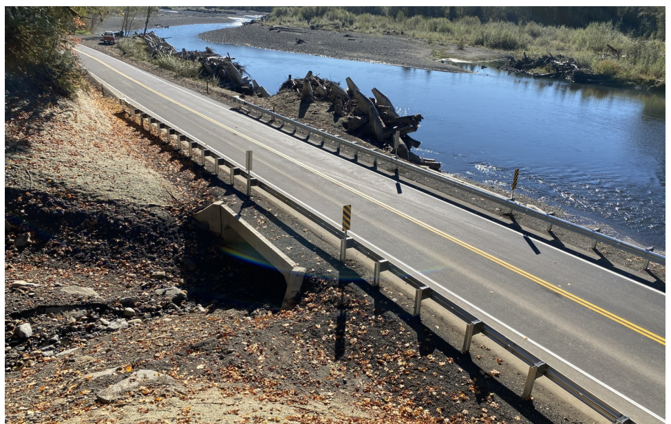
Completed Box Culvert a MP 4.3 of Upper Hoh Road.
