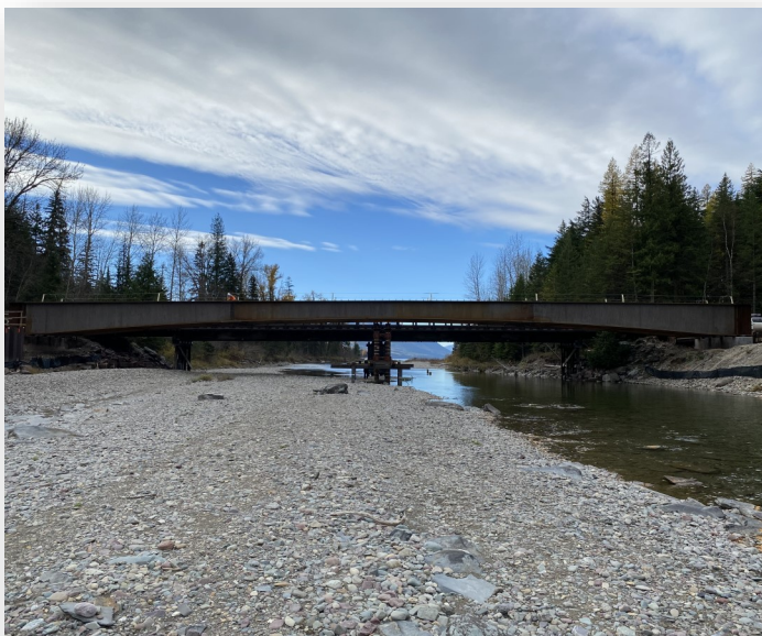
Upstream View of Bridge Superstructure
