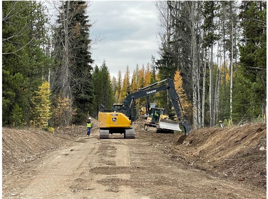
Cutting Ditches at N. fork road
