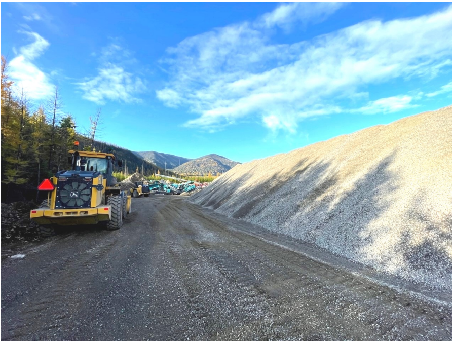
Aggregate Stockpile Produced at Whale Creek Pit
