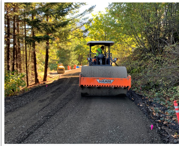
Compacting Aggregate at East Trail
