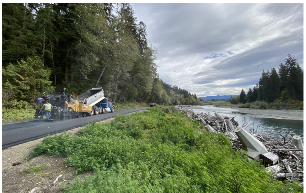
Paving the MP 4 overlay behind the ELJs that were installed in 2022
