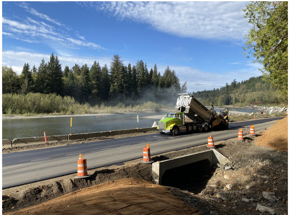
Asphalt paving over the new MP 4 box culvert.
