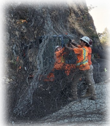
Below: Constructing a temporary rockfall containment net for scaling operations
