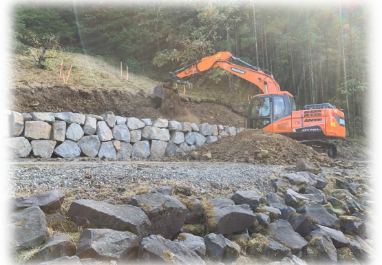
Above: Constructing Rockery Wall at Viento Creek Trailhead
