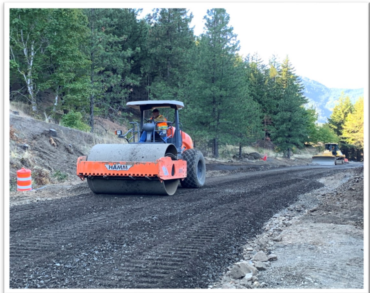
Roadway Aggregate at East Trail
