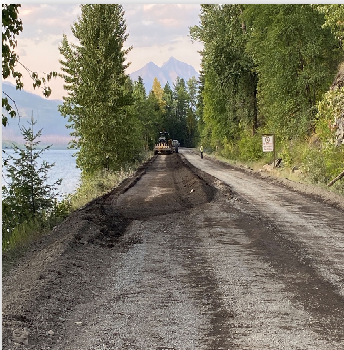
Grading operations on GTSR
