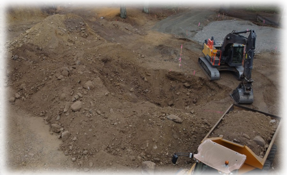
Excavation for sewer septic tank
