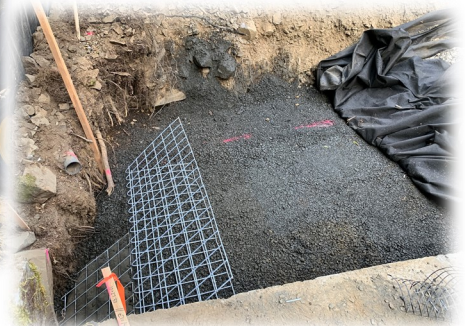
Below: Facing units placed for reinforced soil slope
