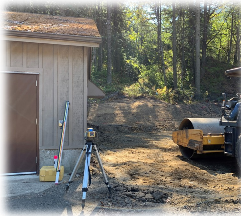
Compacting footing for building expansion
