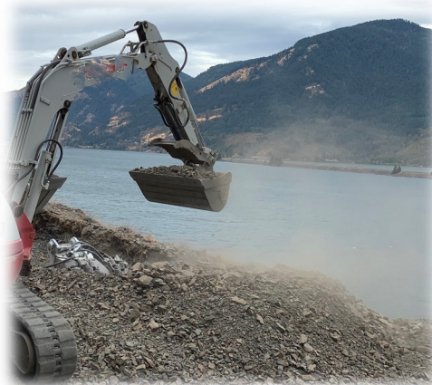
Below left and right: West bench retaining wall foundation excavation
