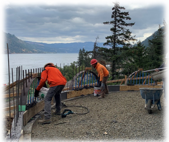
Right: East bench picket base concrete pouring
