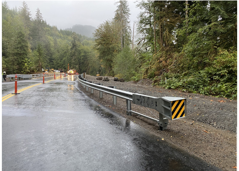
Guardrail installed at the Tower Creek Bridge
