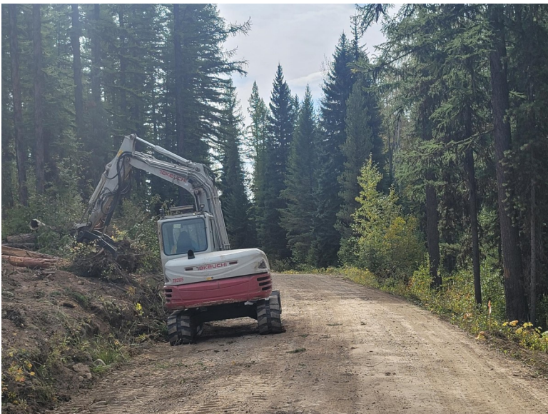
Clearing and Grubbing at N. Fork Rd.
