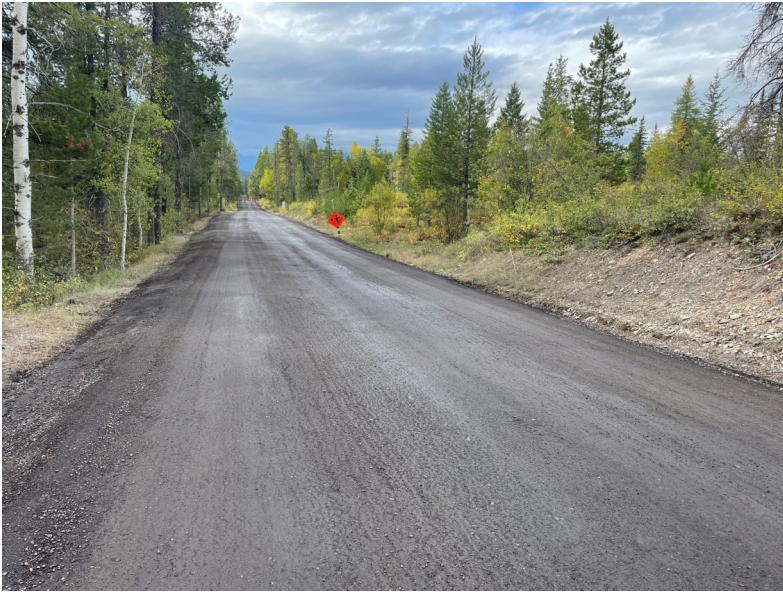
Recycled Asphalt Placed at N. Belton Stage Rd
