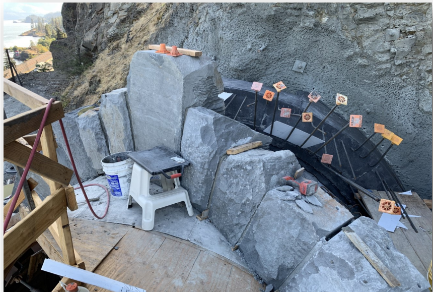
Arch Stone Installation in West Portal
