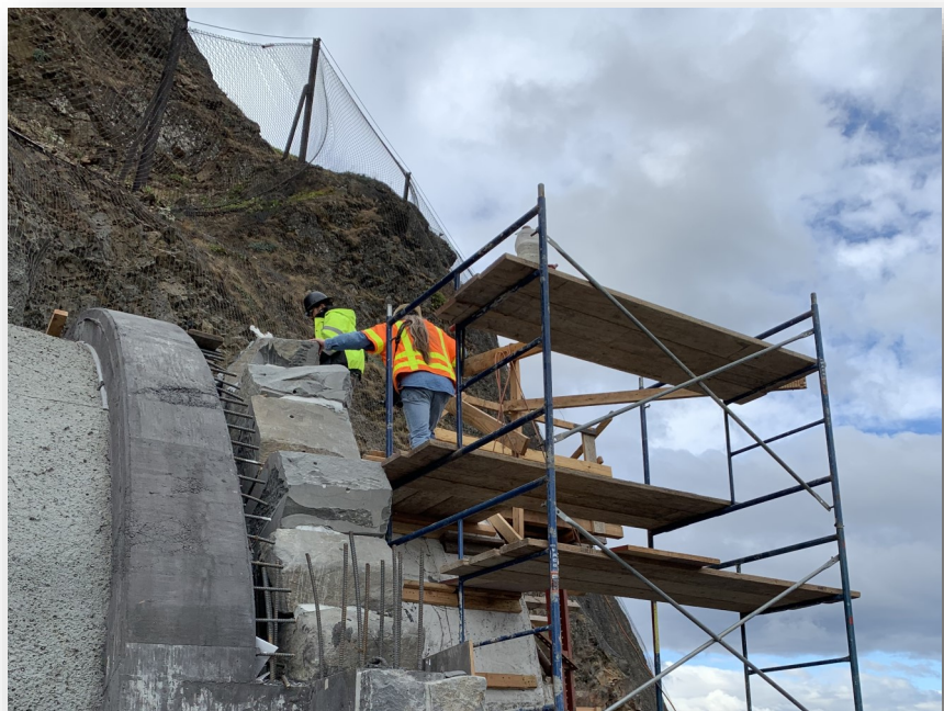
Arch Stone Installation in West Portal
