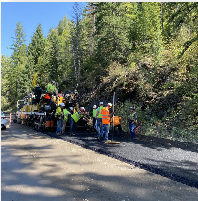
Paving Test Strip on GTSR
