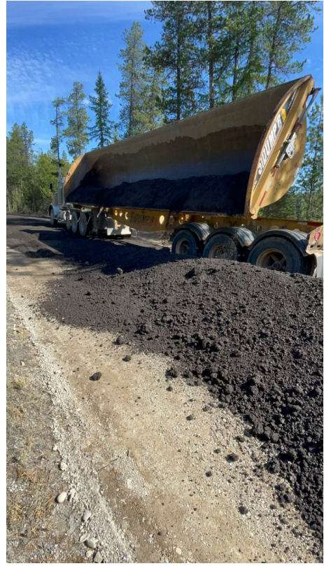
Placing Recycled Aggregate Base on N. Belton Stage Road.
