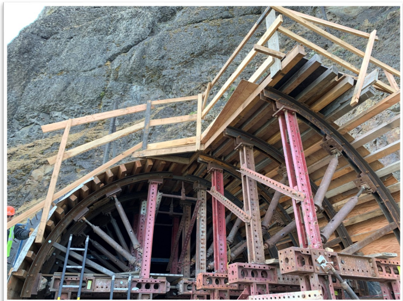
Concrete Structure Support Form at Arch
